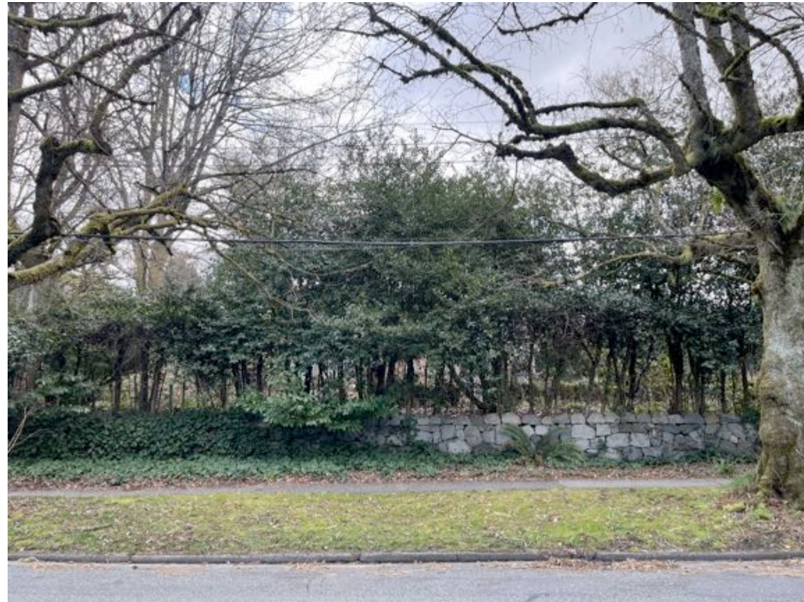
INTACT PORTION OF EXISTING WALL. HOLLY HEDGE BEHIND.
