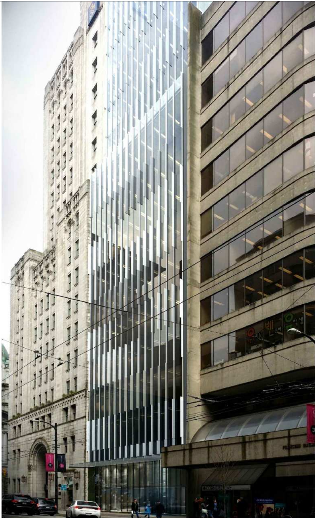
1 View Looking West Down W Hastings St. N.T.S.
