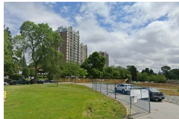
4- View from West
