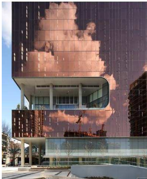
Figure 2: Existing Building from the West
