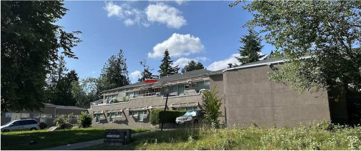
SALVATION ARMY HOMESTEAD - 975 WEST 57 th AVENUE
