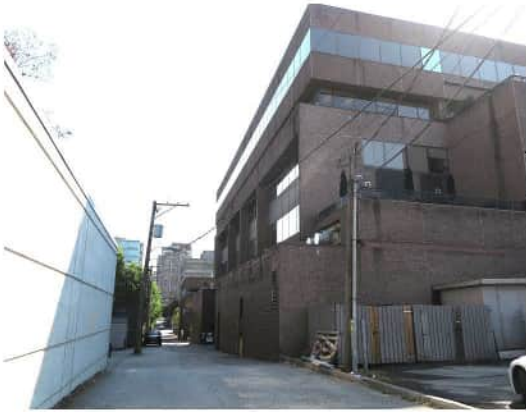
LANE - LOOKING EAST
