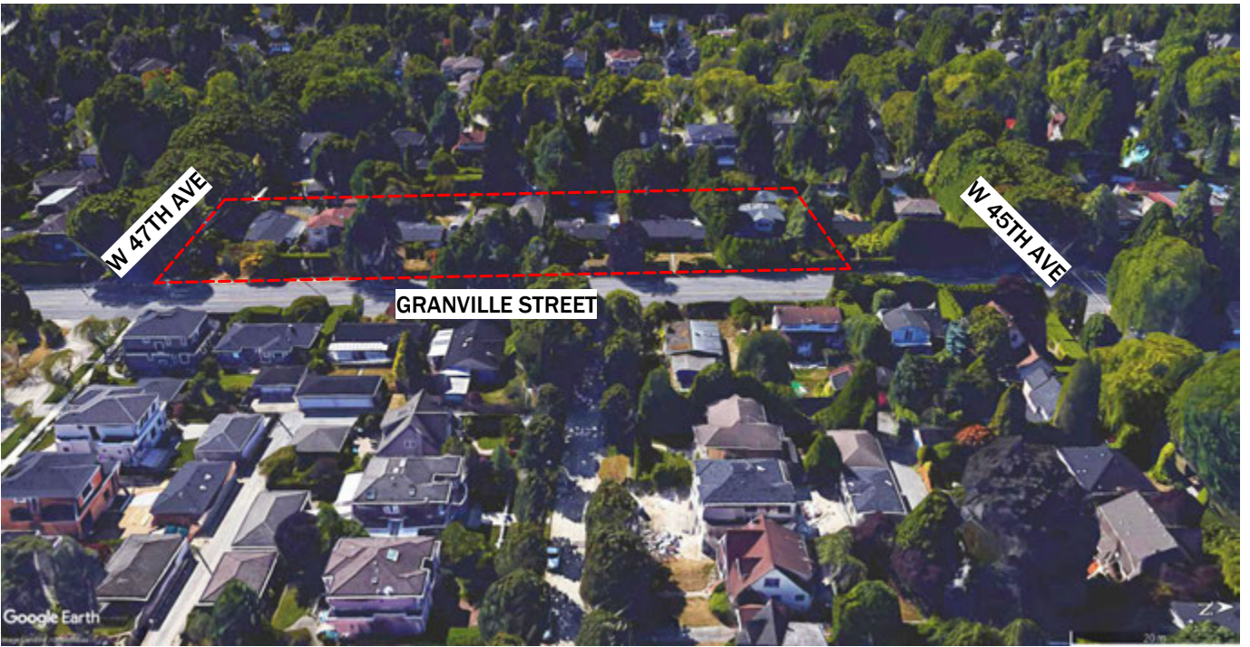
AERIAL VIEW LOOKING WEST
