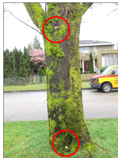
April 6/17 - Tree #124 - Fungal activity (REMOVED)
