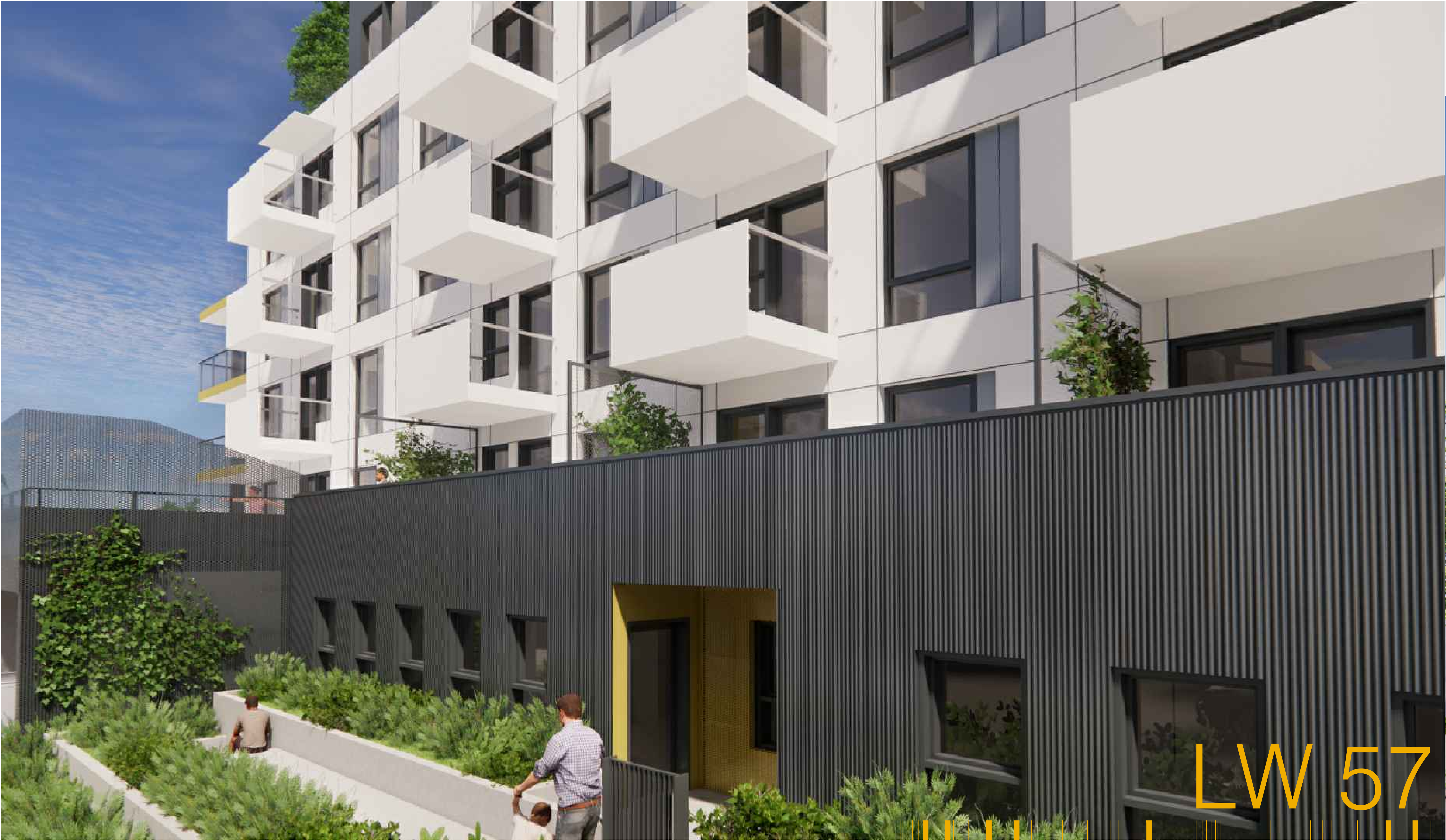
VIEW LOOKING WEST AT THE GROUND LEVEL UNITS partial south elevation
