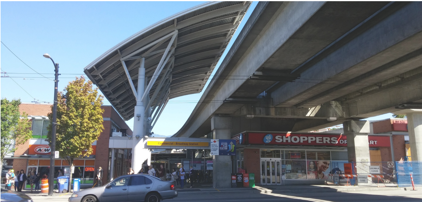
C. COMMERCIAL/ BROADWAY SKYTRAIN STATION
