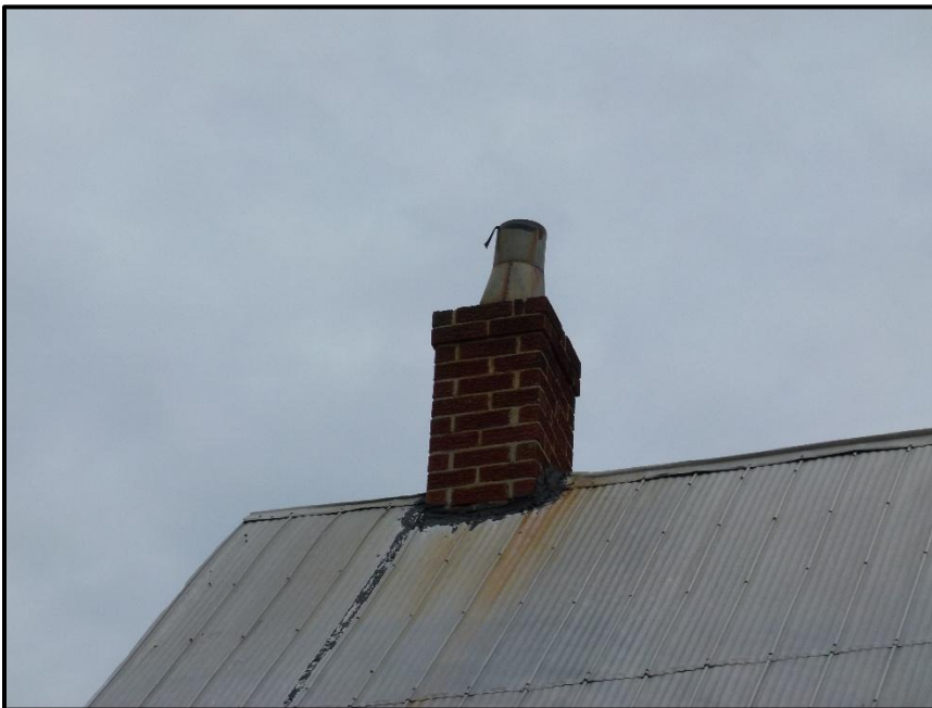
Photograph 26: A close-up of the metal cap on the chimney of Building #3 (April 21 st , 2025).
