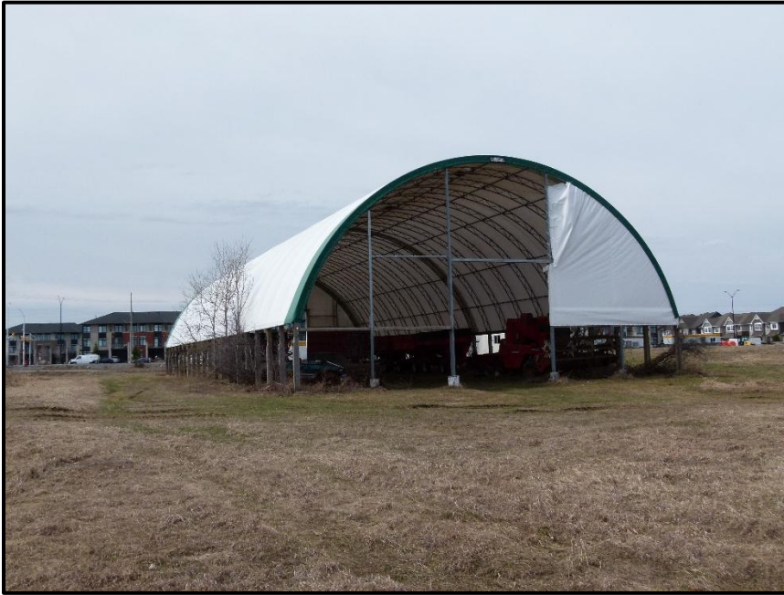
Photograph 23: Looking west at Building #1. No evidence of Barn Swallow nesting was observed within Building #1 (April 21 st , 2025).
