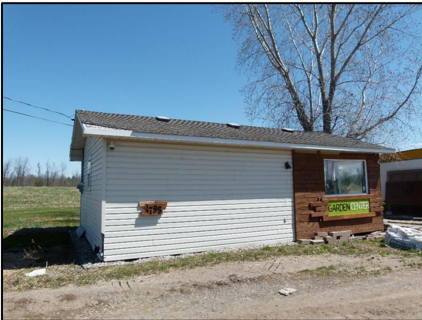
Photograph 24: Looking east at Building #2. No evidence of Barn Swallow nesting was observed within Building #2 (April 28 th , 2025).
