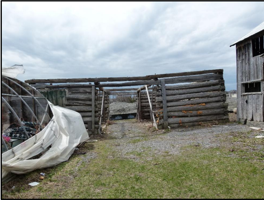
Photograph 31: Looking west at Building #7. No evidence of Barn Swallow nesting was observed within Building #7 (April 21 st , 2025).
