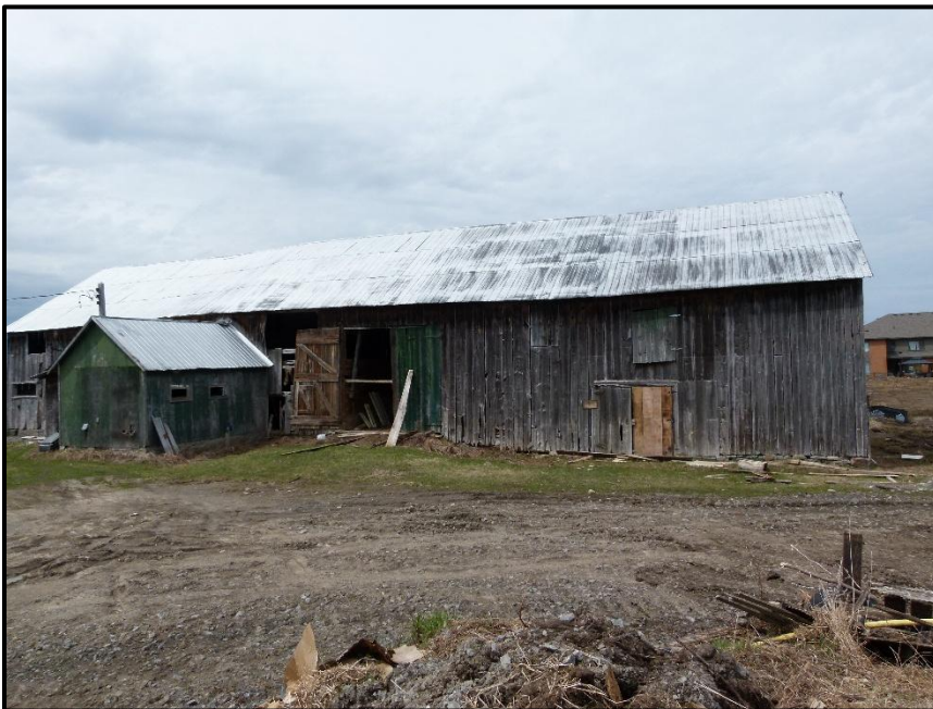
Photograph 32: Looking north at Building #8. Active Barn Swallow nests were observed within Building #8 (April 21 st , 2025).
