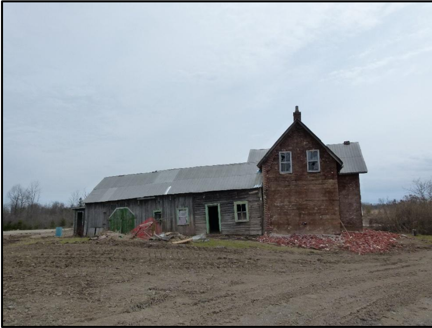
Photograph 25: Looking south at Building #3. Active Barn Swallow nests were observed within the garage/workshop attached to the farmhouse (April 21 st , 2025).
