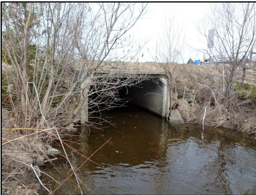
Photograph 18: Looking upstream at the large box culvert under the driveway that leads to the old farmhouse (April 21 st , 2025).
