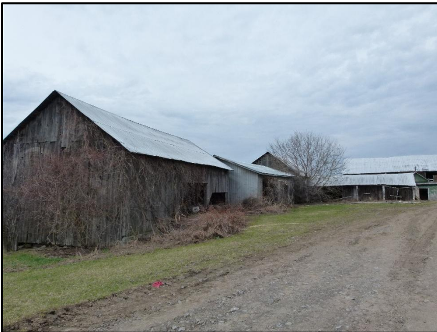
Photograph 28: Looking northwest at Building #5. Active Barn Swallow nests were observed within Building #5 (April 21 st , 2025).
