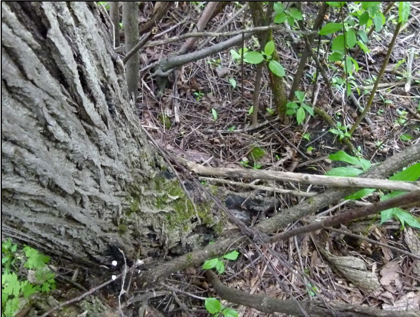
Photograph 16: Butternut Tree #7 – assessed as Category 1 (non-retainable). Extensive canker is visible on the root flare (May 23 rd , 2025).
