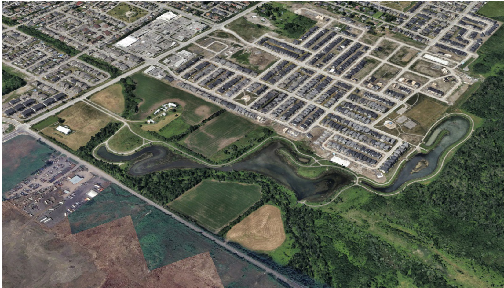
View of Existing Findlay Creek Stormwater Management Facility
