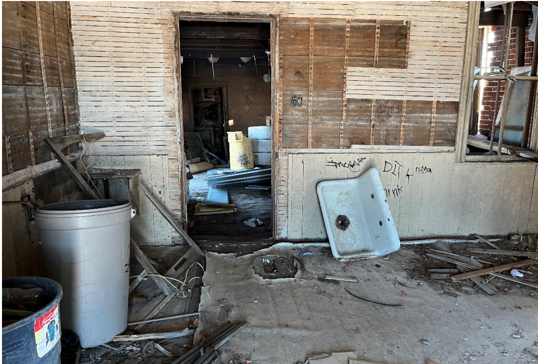
Photograph 3: First floor interior of the farmhouse.
