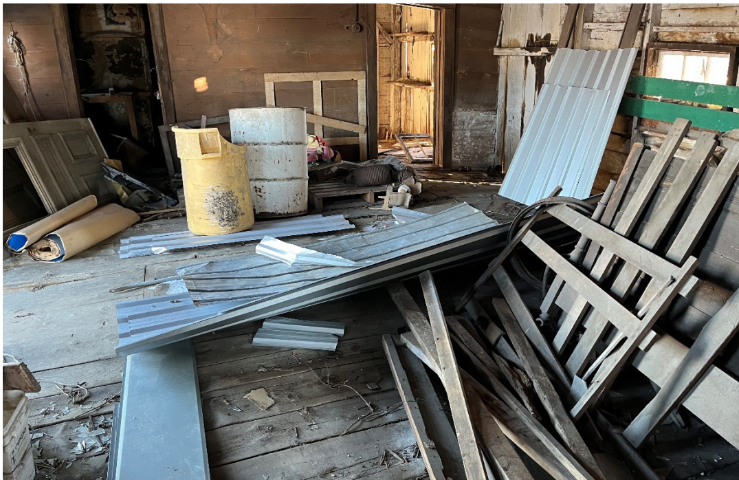
Photograph 4: View of interior of the addition to the farmhouse.
