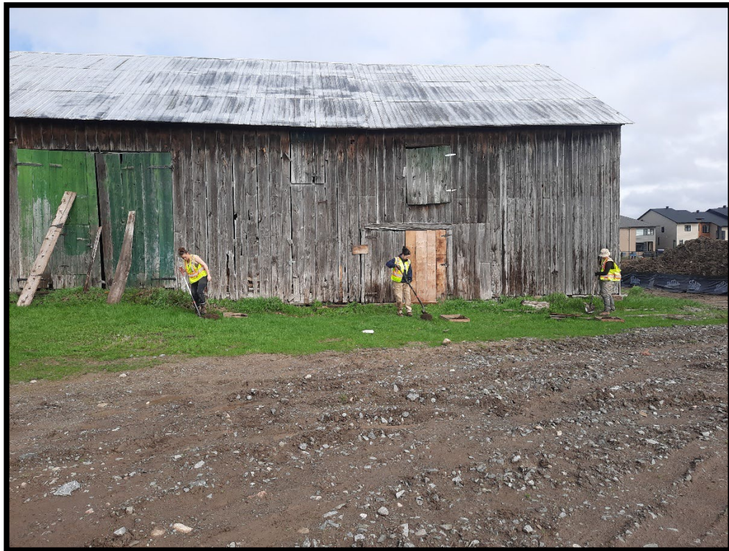
Figure 26: Test pitting in progress (MH1366-D009).
