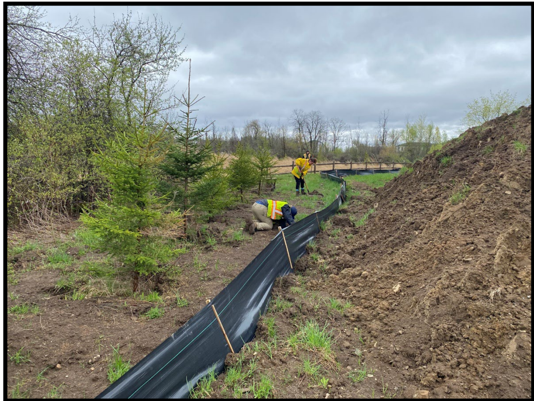
Figure 30: Test pitting in progress (MH1366-D077).
