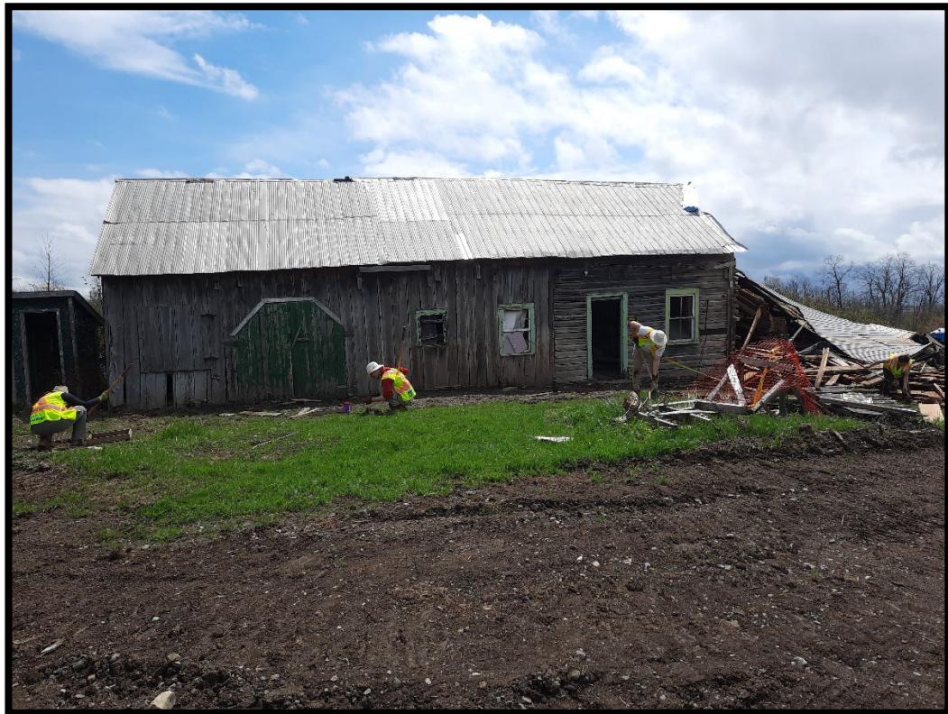
Figure 28: Test pitting in progress (MH1366-D031).
