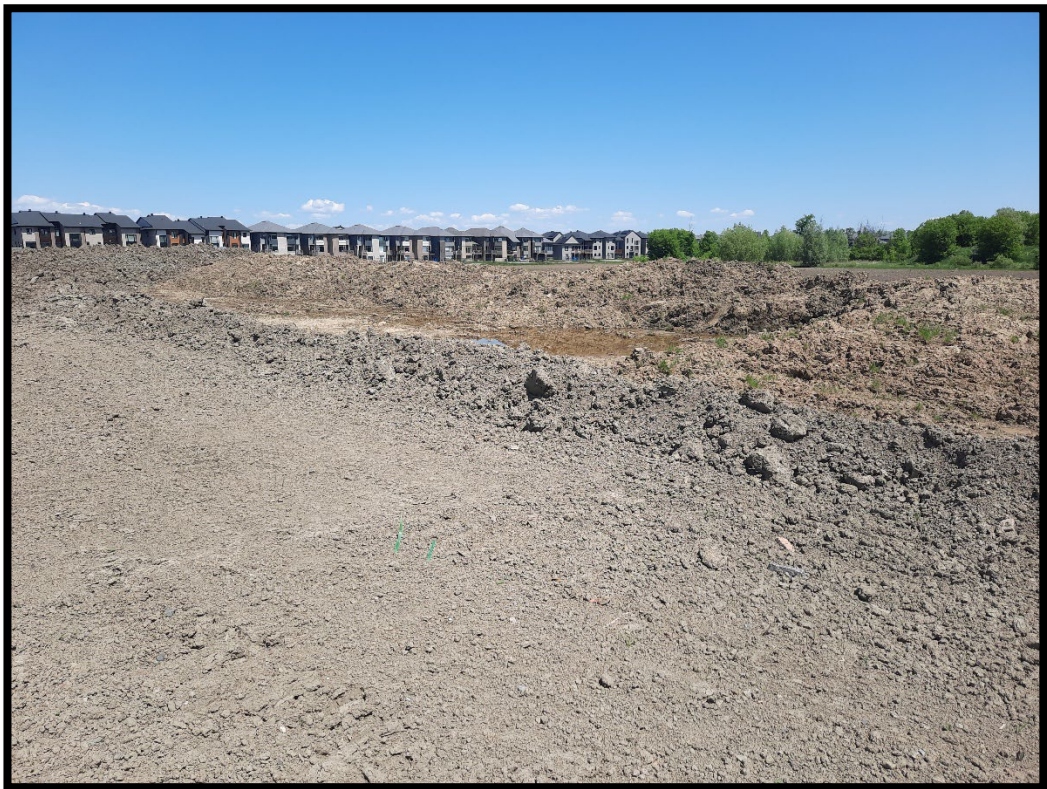
Figure 10: Example of disturbed conditions (MH1366-D151).
