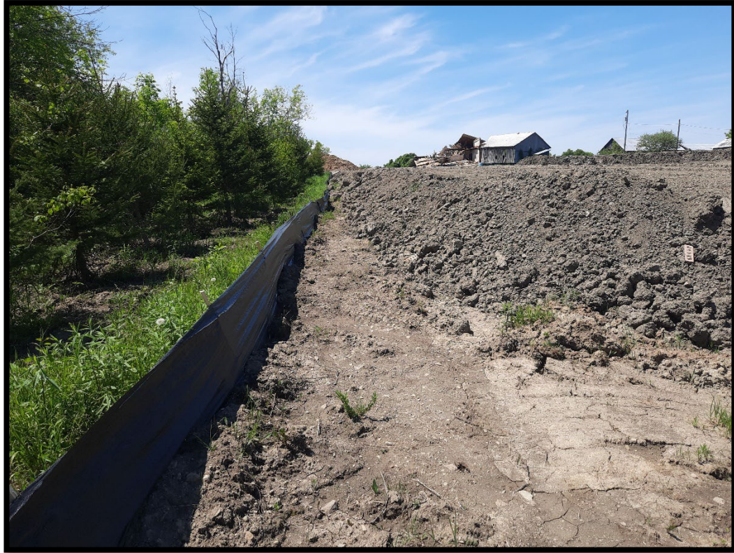
Figure 11: Example of disturbed conditions (MH1366-D153).
