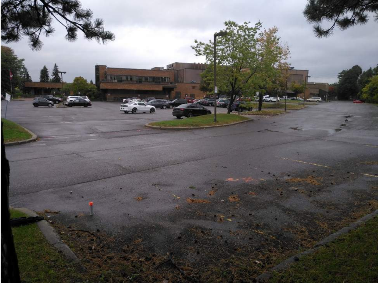
Photo 22: View of subject property from southwest corner of the parking area, facing northeast
