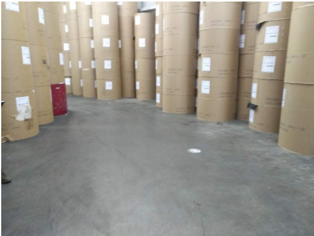
Photo 17: Paper storage area and existing monitoring well
