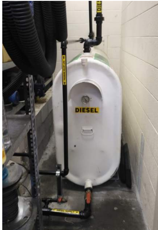
Photo 4: Diesel AST and part of brick enclosure
