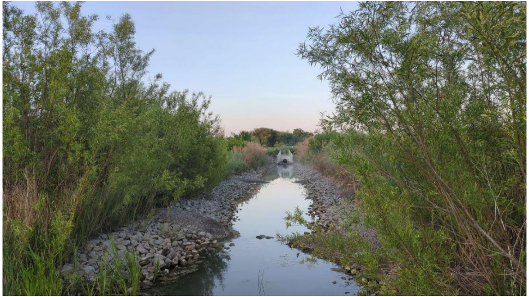
Photo 7: Drain from stormwater management pond leading to Carp River 9 June 16, 2025).
