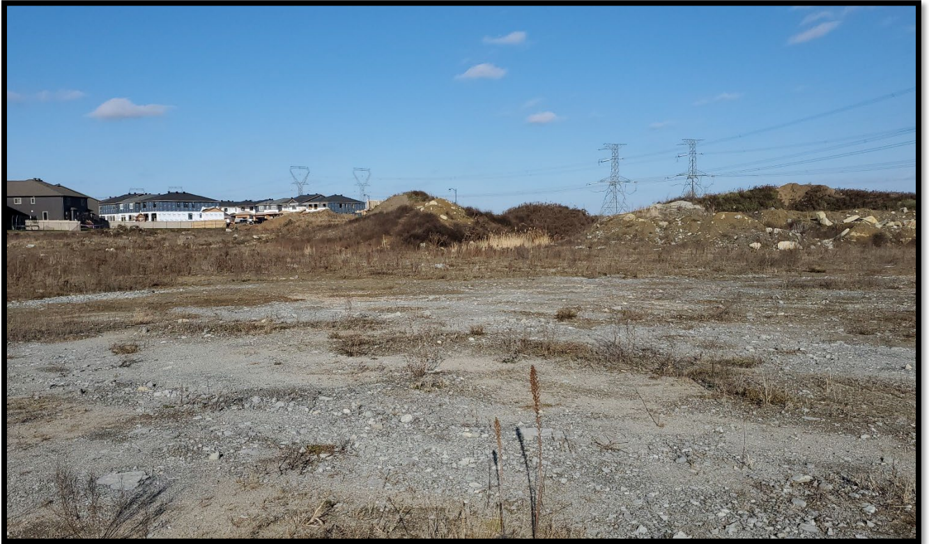
Figure 19: Stripped and disturbed gravelly area (MH1066-D17).
