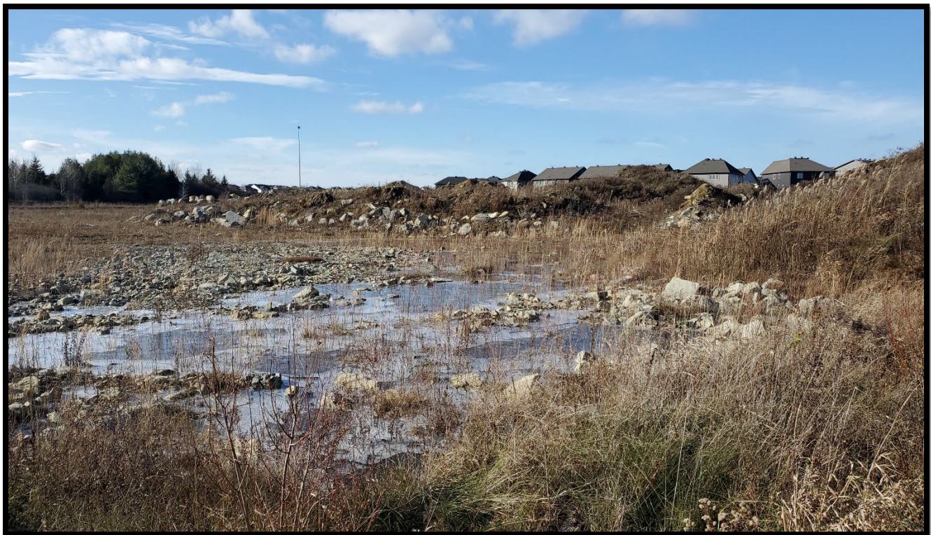
Figure 18: Stripped area and earth stockpiles (MH1066-D13).
