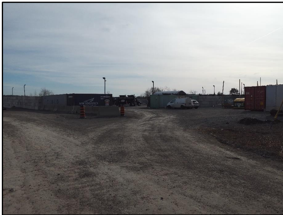
Image 14. View of construction site at the centre of the study area, facing northeast. (PR23-082D188)
