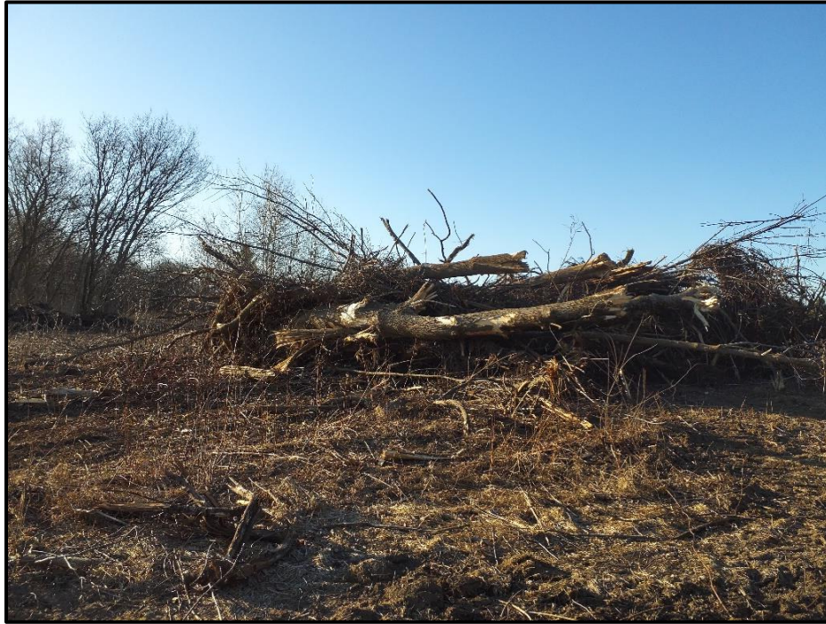
Image 3. View of cleared woodlot showing remaining brush piles, facing southeast. (PR23-082D007)
