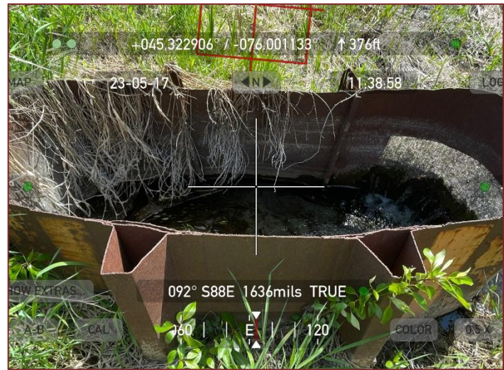
Site Photograph 6: The vertical drain on-site.
