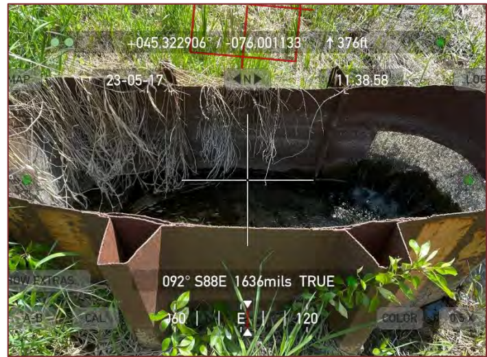
Site Photograph 6: The vertical drain on-site.
