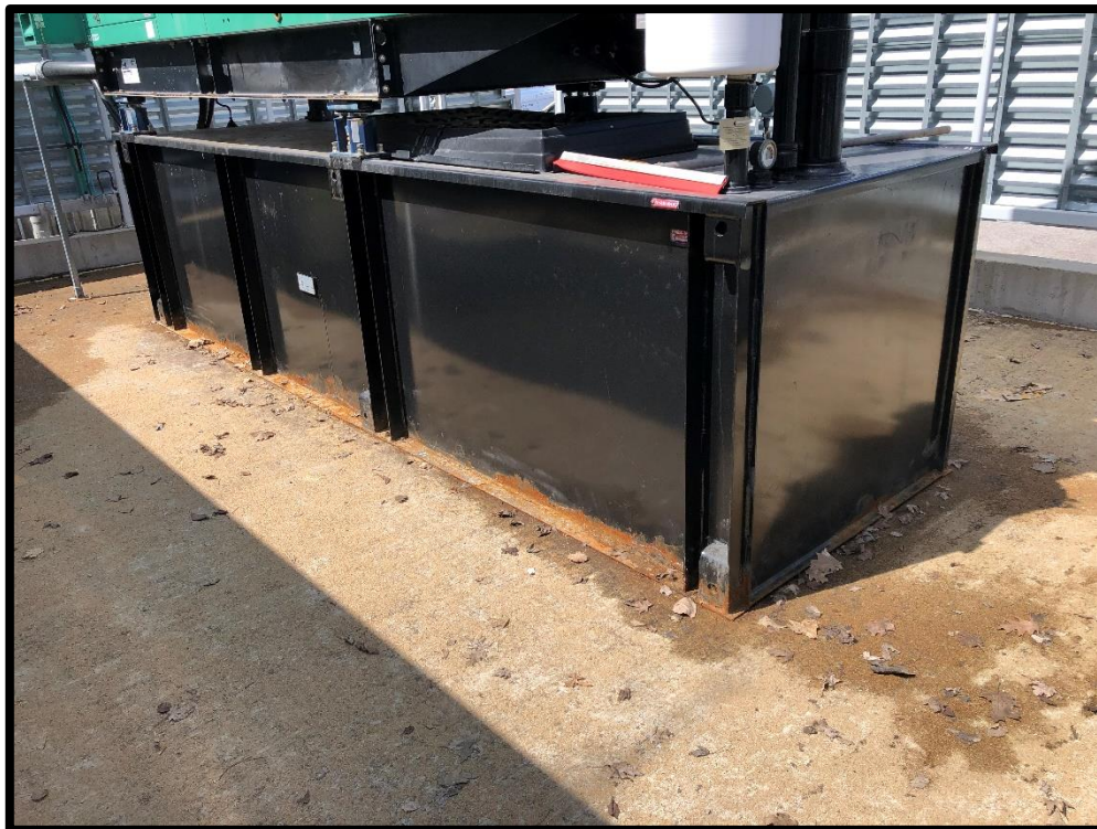
Photograph 4: View of the AST on the northeast corner of the Brooke Claxton building, facing south.
