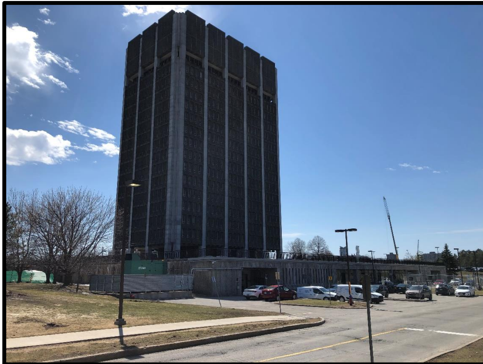
Photograph 2: View of the back of the Brooke Claxton building, facing south.
