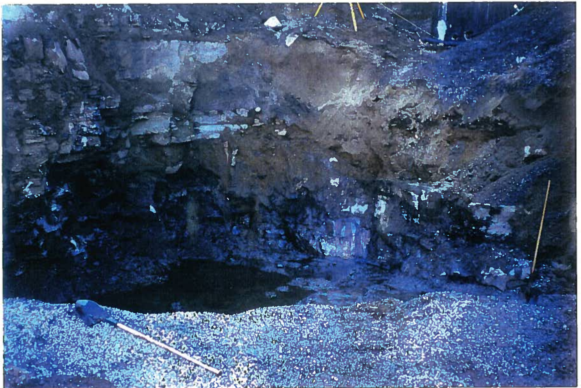
PHOTO 2 Southwest corner of excavation.
