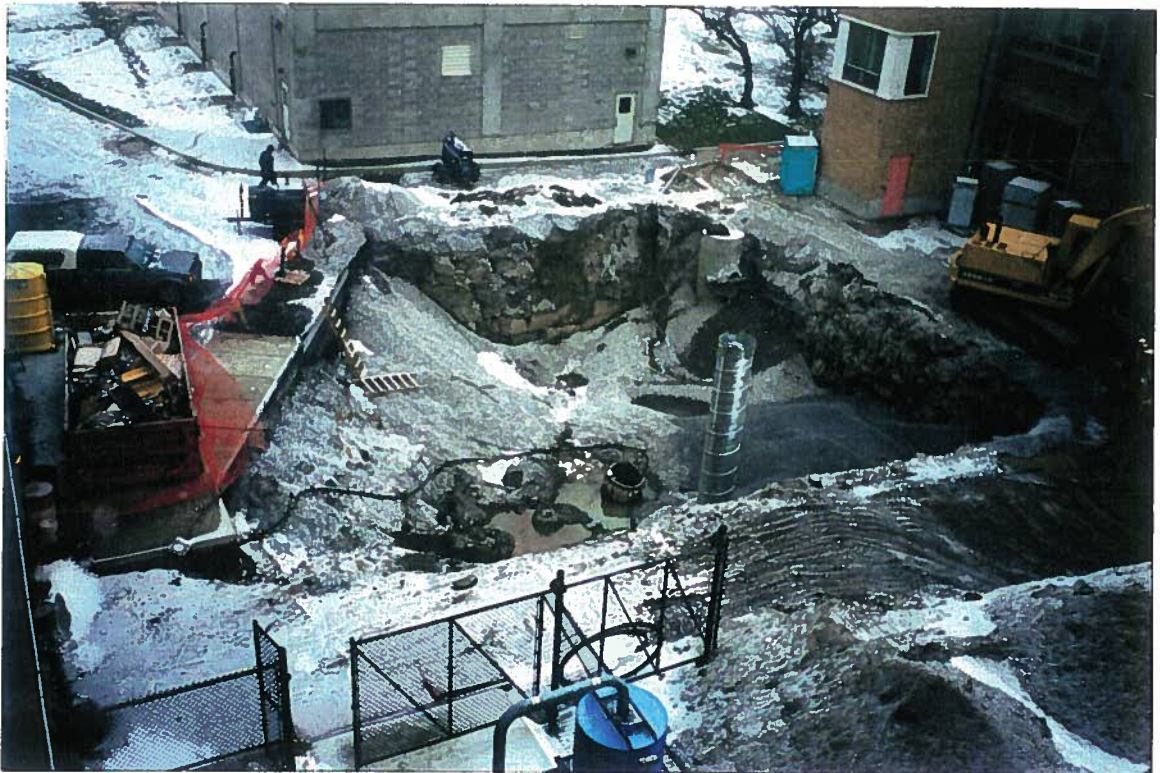
PHOTO 4 Excavation after tank removal.
