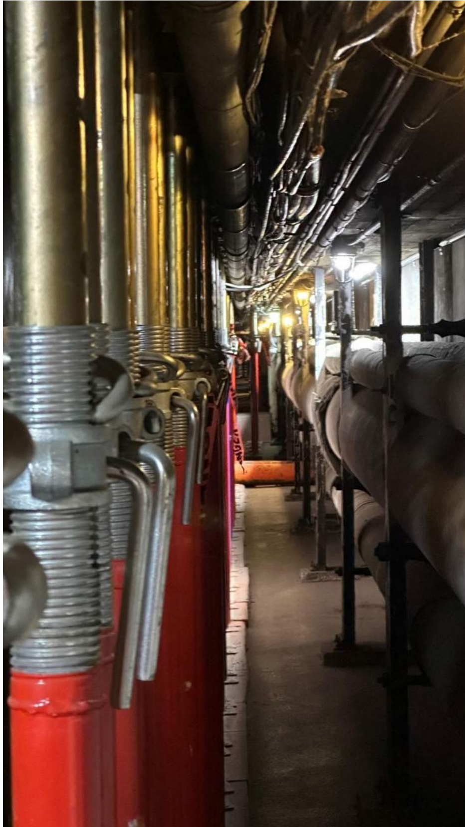
Image H.6: Tunnel System – Current Condition Throughout
