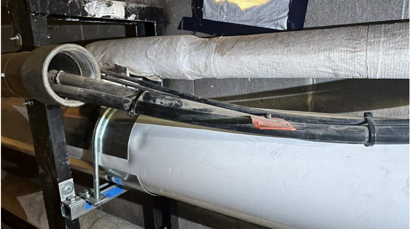
Image H.22: Standards Building – Tunnel System Entry Into Building
