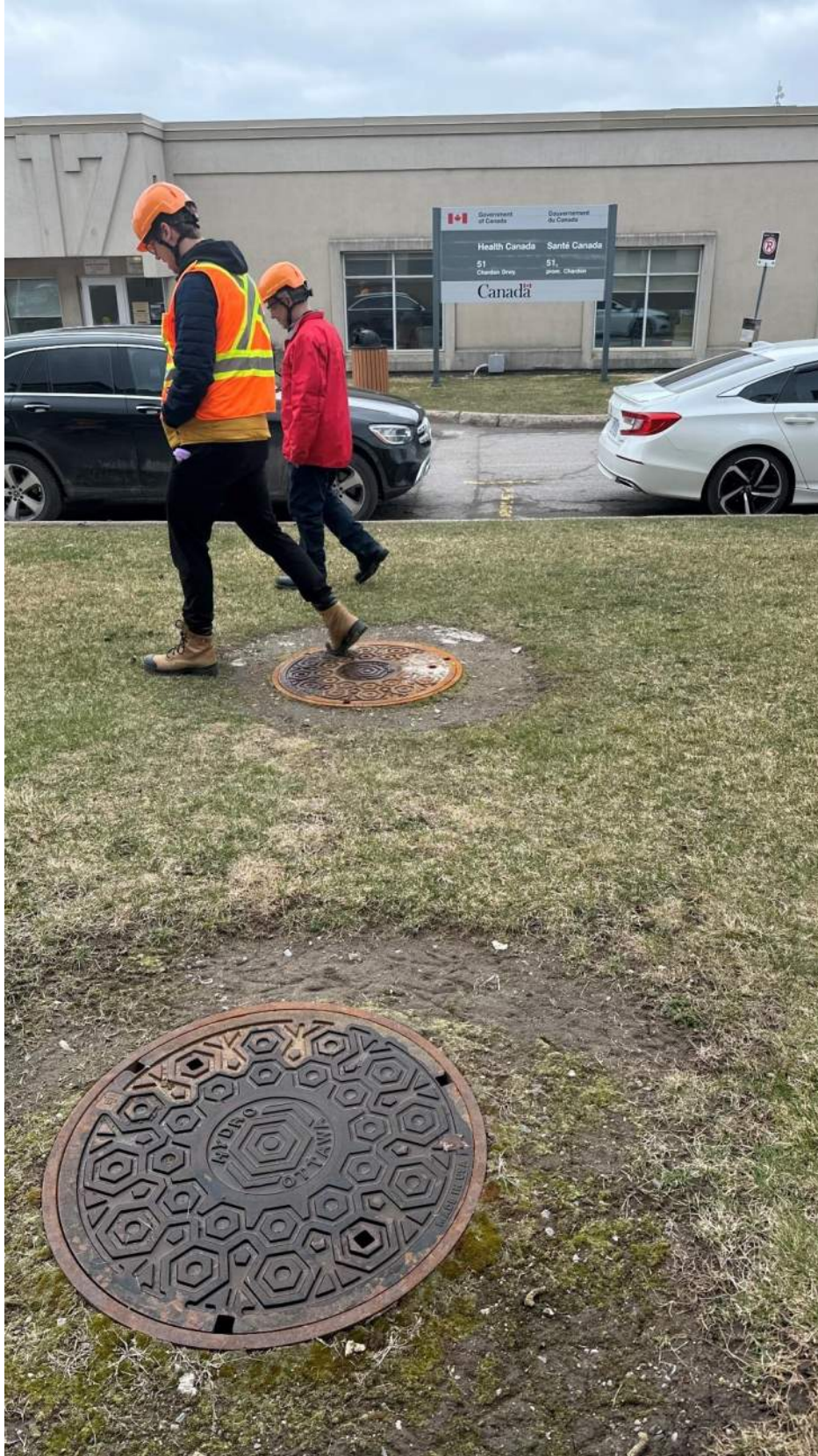
Image H.4: Heating & Cooling Plant – Duct Entry, West Side Exterior
