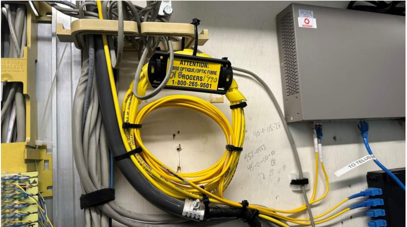
Image H.9: Personnel Records Building – Rogers Presence
