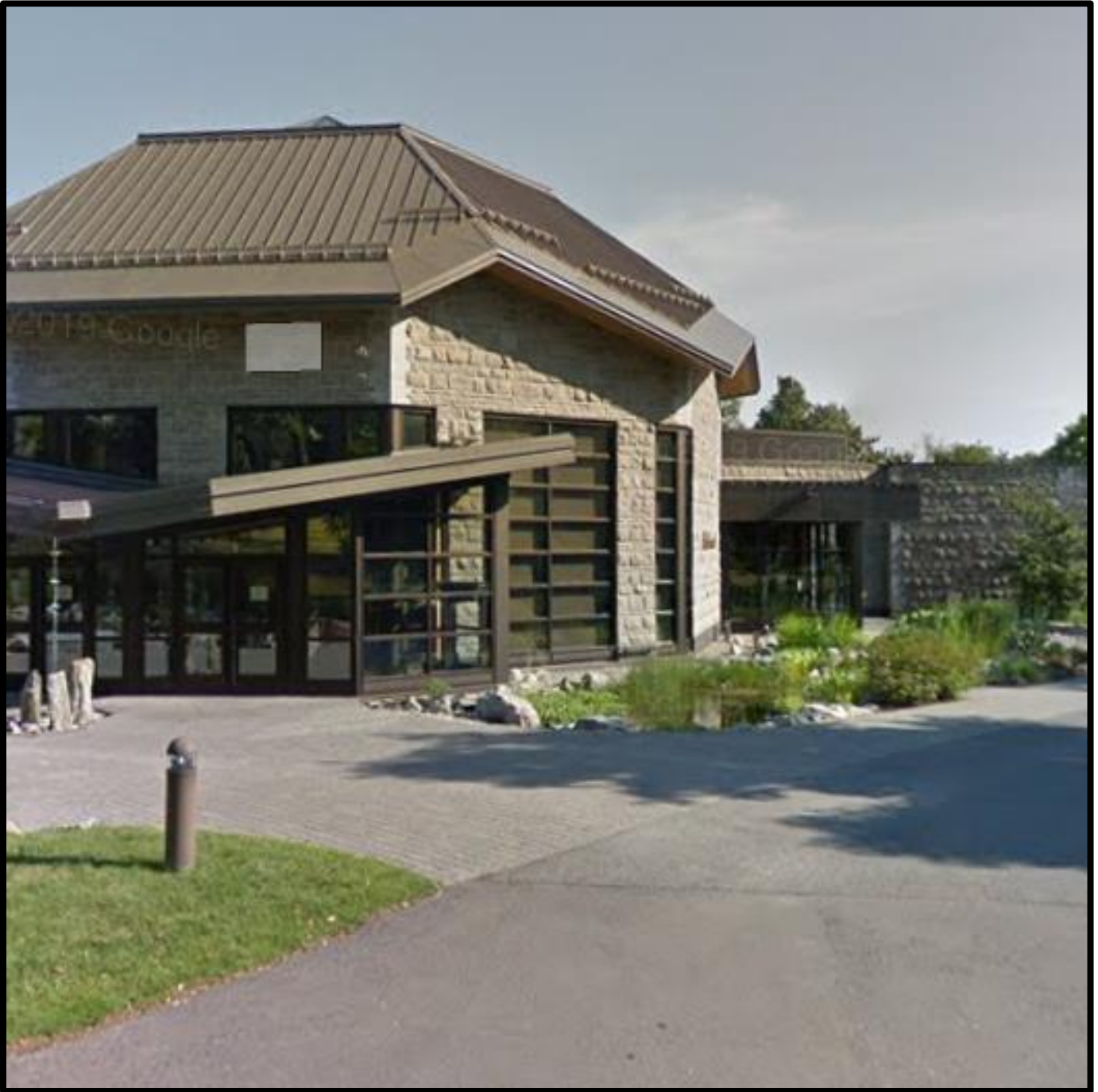
Photograph 1: View of the new building section, facing south.
