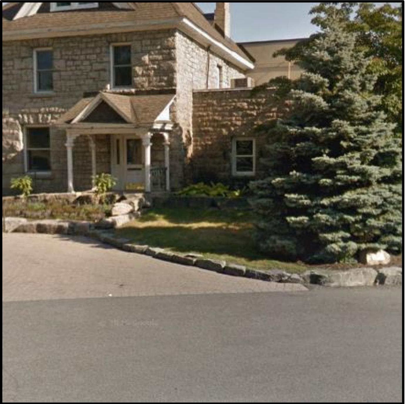
Photograph 2: View of the old building section, facing south.
