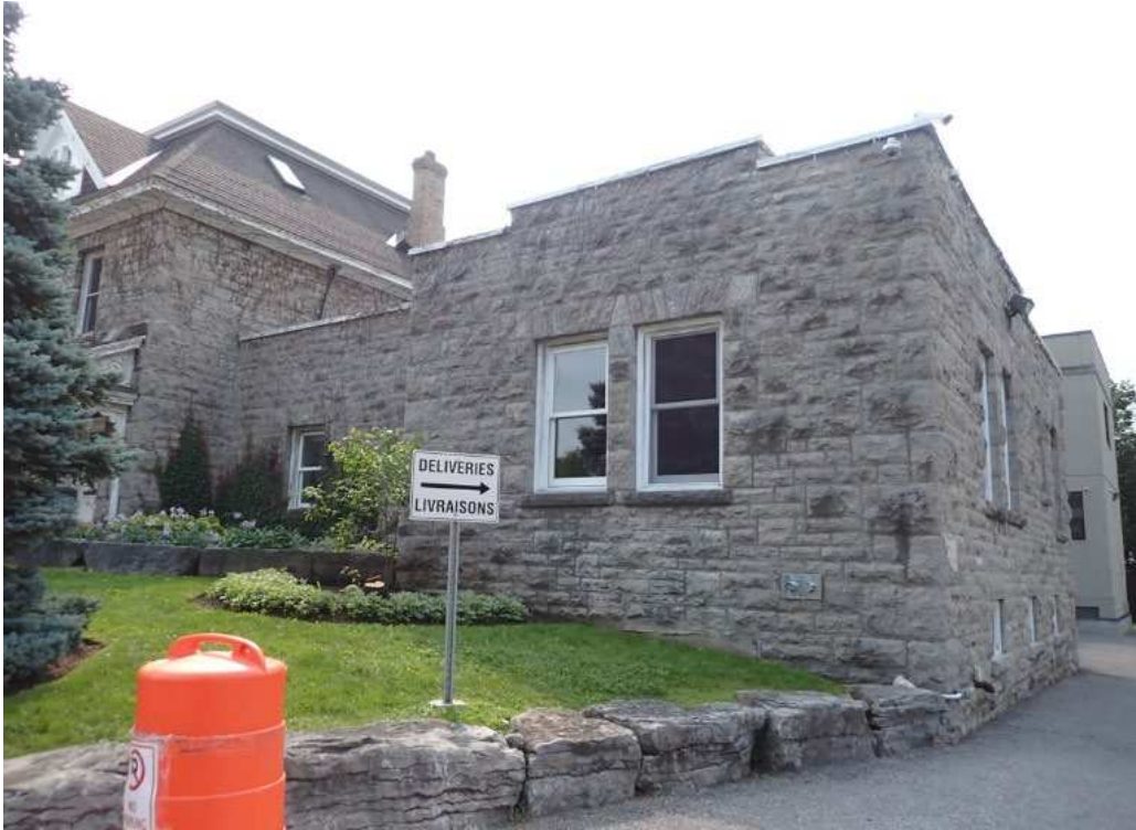
Figure 9: Existing addition west of the Stone Residence (Source: RMA+SH architects, 2026).
