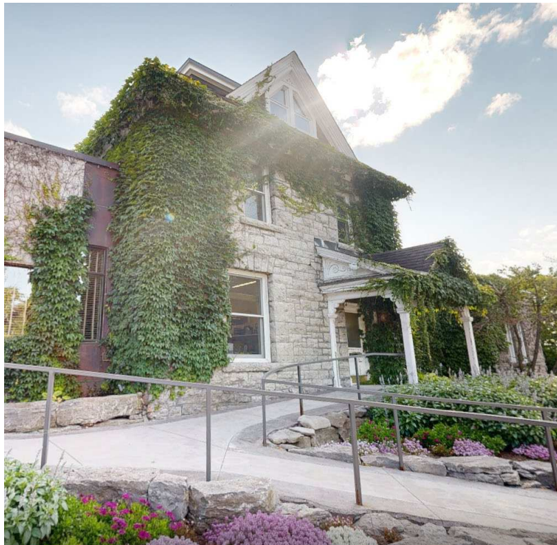
Figure 1: The Stone Residence from its principal north façade, note heavy vine growth (Source: RMA+SH architects, 2026).
