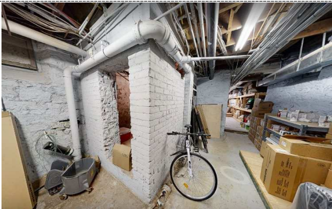
Figure 16 – Stone Residence Basement mechanical room. Note painted brick and limestone foundation walls.
