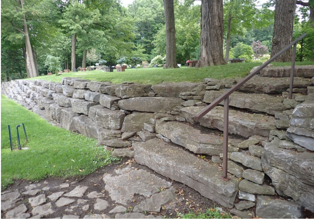
Figure 10: Example of limestone use throughout the cemetery (Source: RMA+SH architects, 2026).
