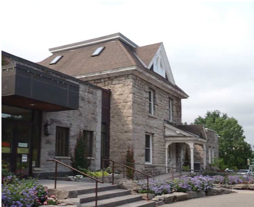
Figure 8: Existing roof on the Stone Residence (Source: RMA+SH architects, 2026).
