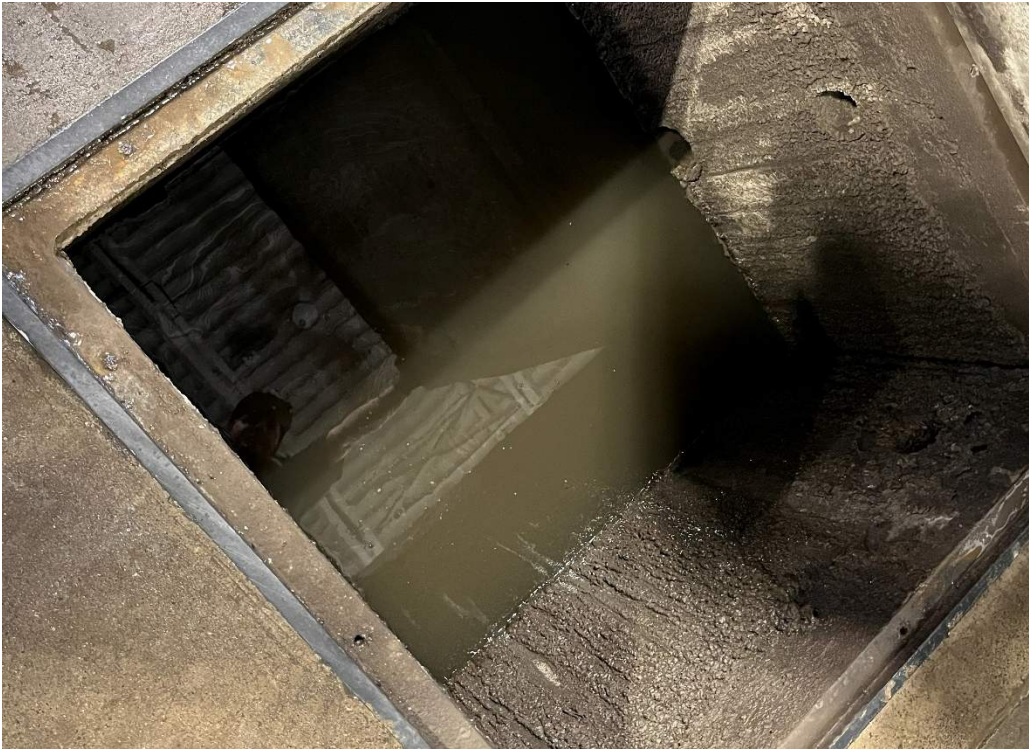
Photograph 5: Interior of the oil/water separator.
