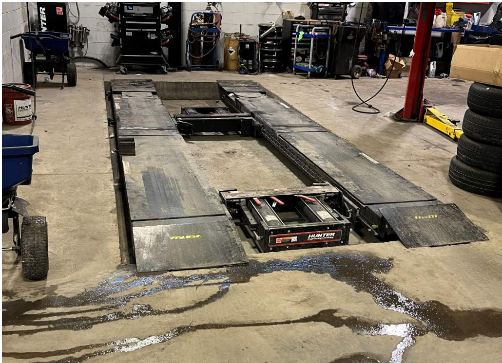
Photograph 2: Service bay with a vehicle alignment rack.
