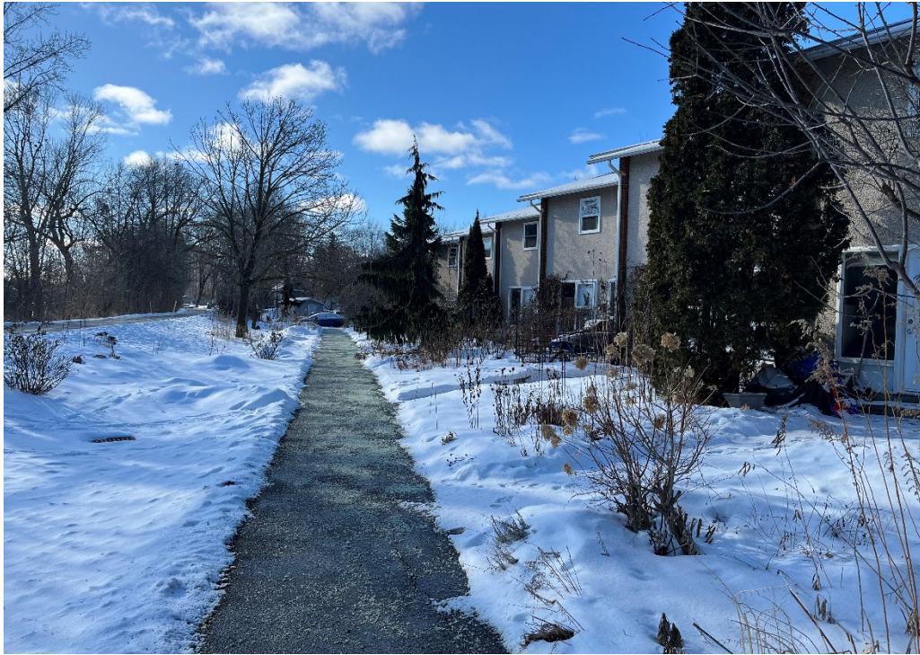
Photograph 1: View looking south, along eastern property limits of the subject site.
