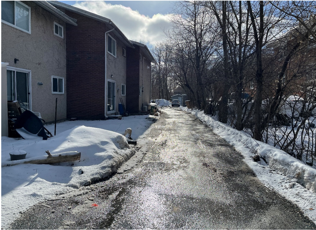
Photograph 3: View looking south, down and across the subject site.
