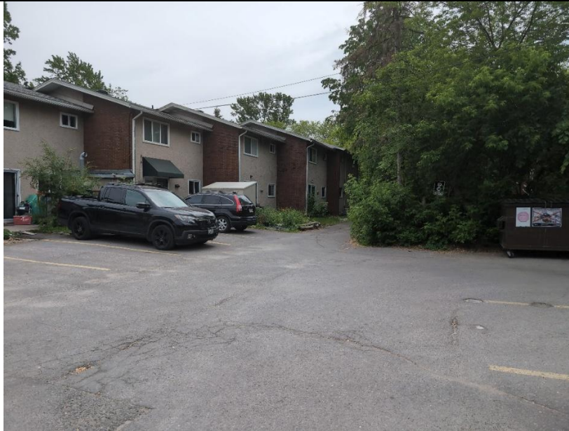
Figure 3 Central paved parking area surrounded by townhomes in the Low Density Residential (CVR_1) unit (photo taken June 5, 2026)
