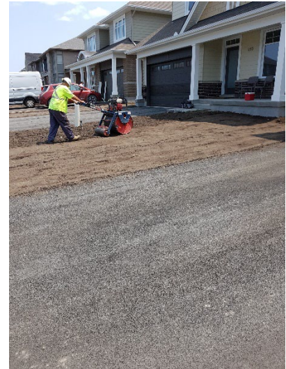
Figure 6.3 Example Soil Amendments – Wateridge Village Phase 1A
