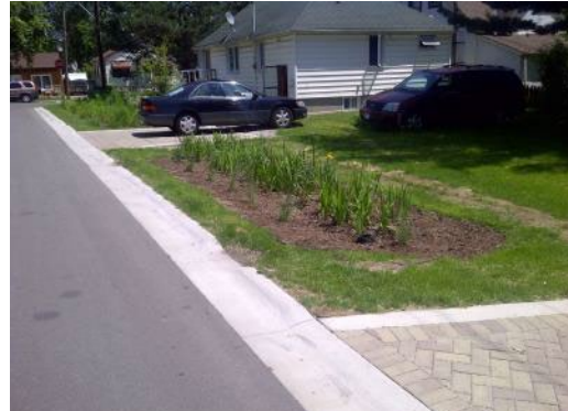
Figure 6.2 Example Bioswales - Mississauga, ON
