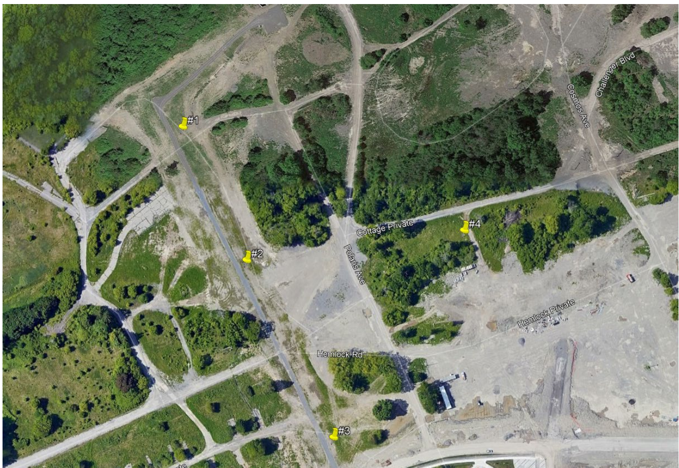
Figure 6.1 2019 In-Situ Infiltration Locations
