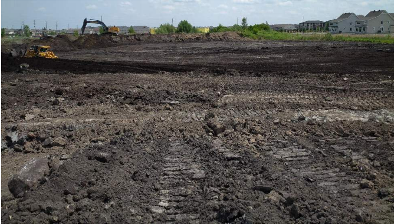
Photograph No. 3: Deepest Part of Removals, Facing East Across Site Over Work Area
