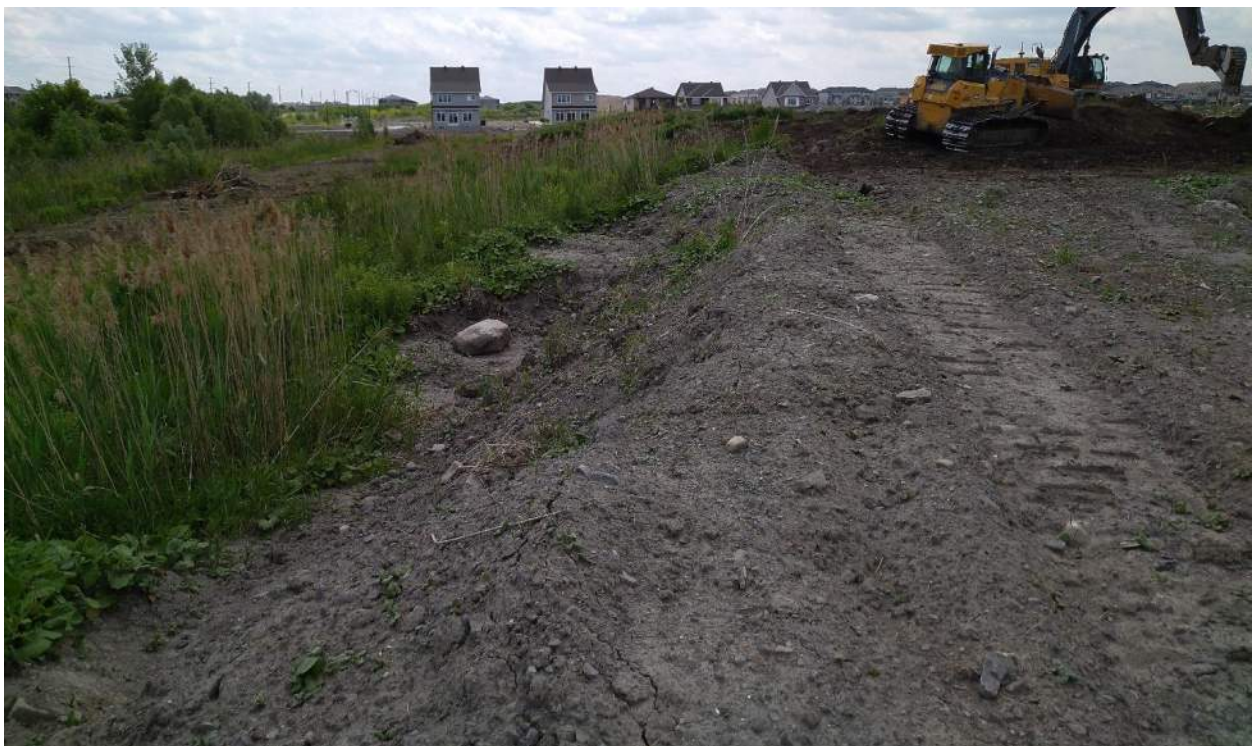
Photograph No. 6: East Edge of Site Facing South
