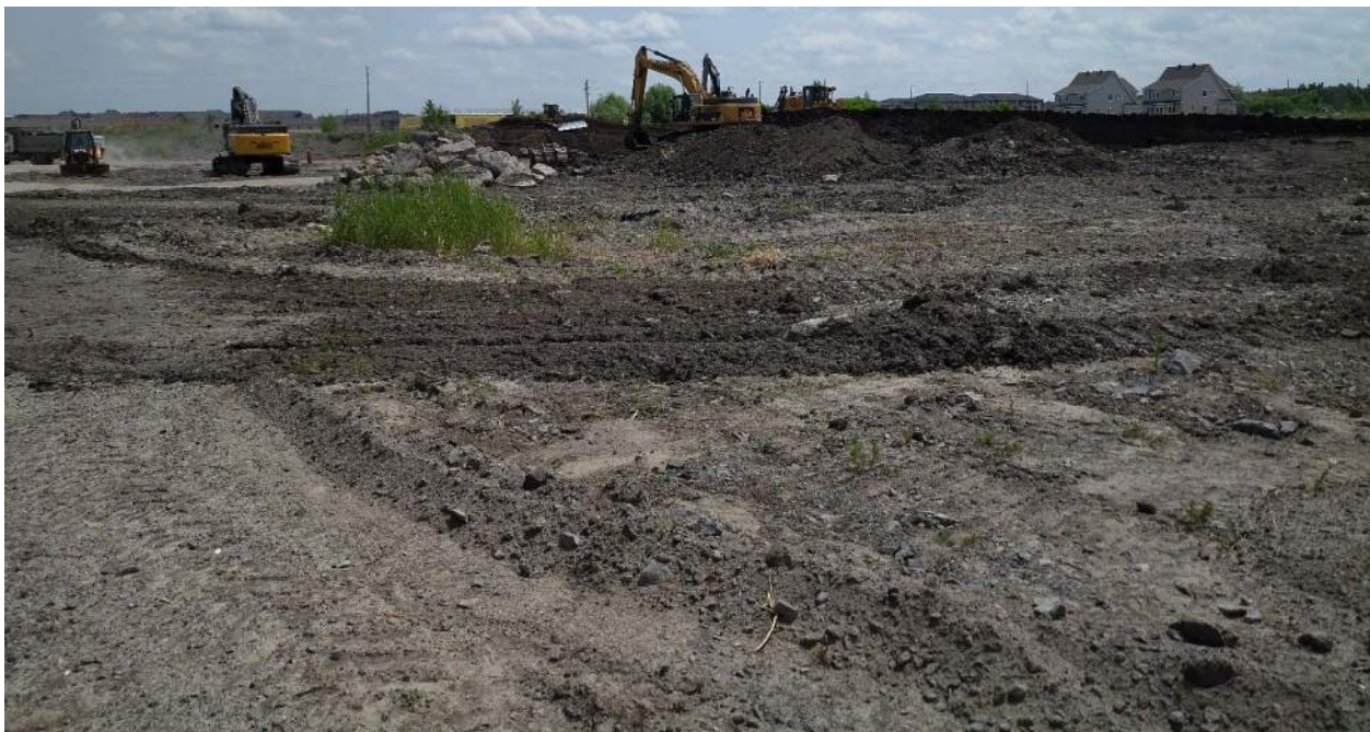
Photograph No. 2: Boulders Also to be Removed
