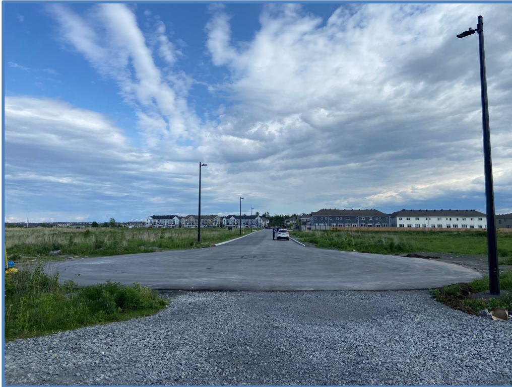
Figure 5: View from End of Culdaff Road
