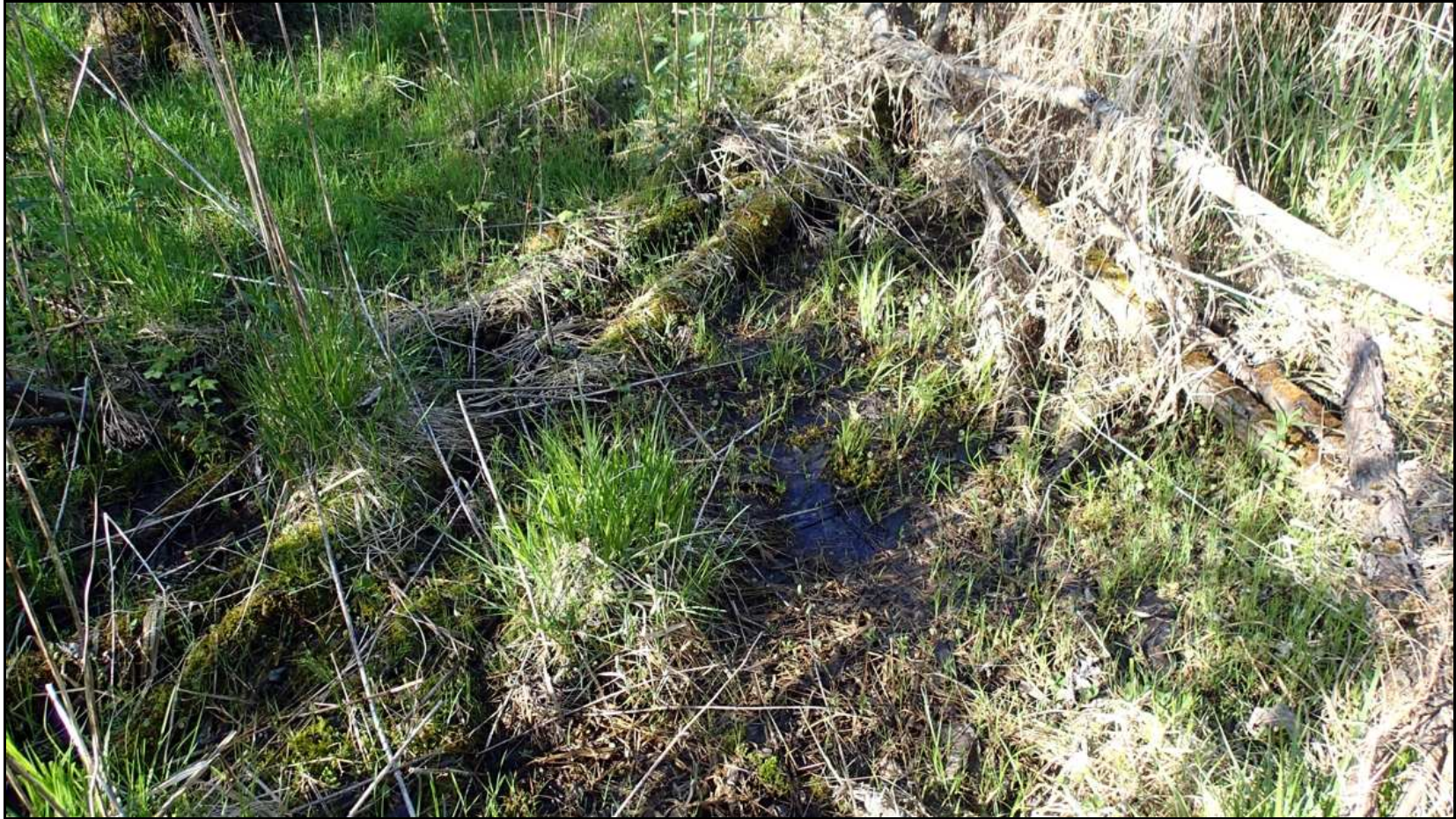
Plate 16: A large section of the northwest corner of the property was unstable wet land with a high water table and alders and reeds.
