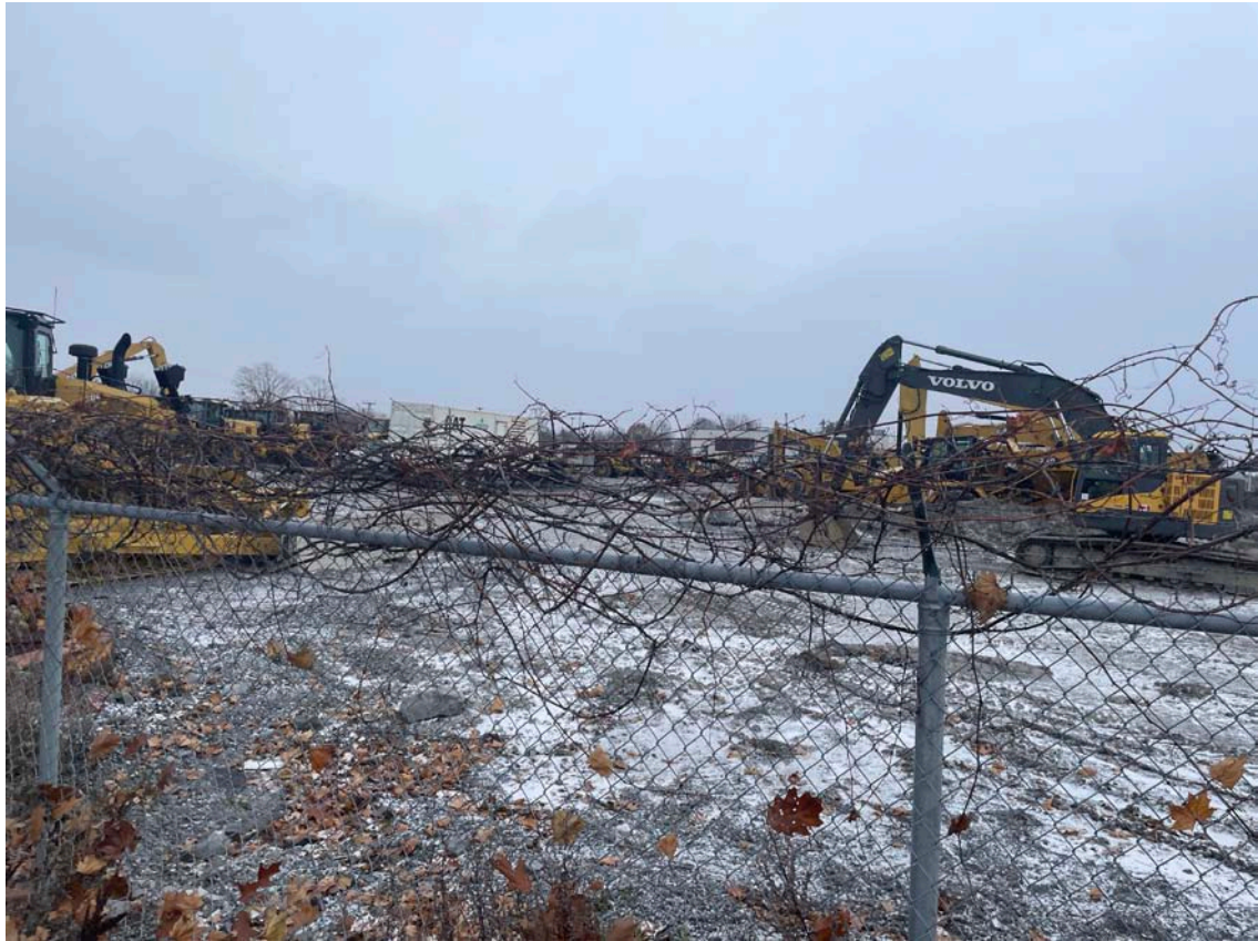
View of site located south of site
