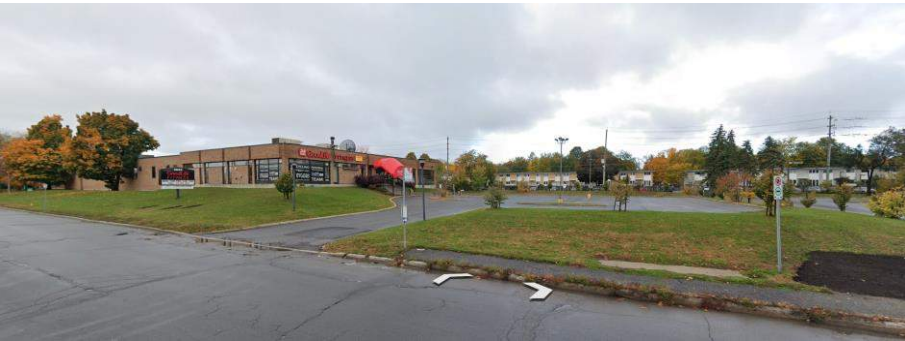
View 2: Looking Northwest @Queensview Drive
