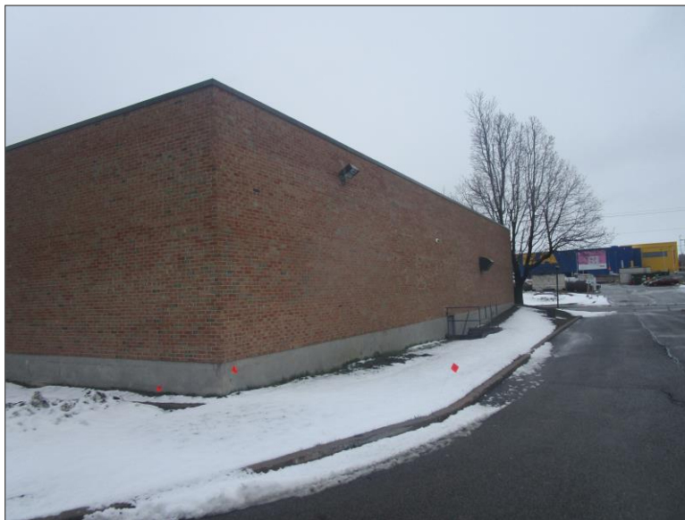
Photo 4 – Site Building (west elevation).
