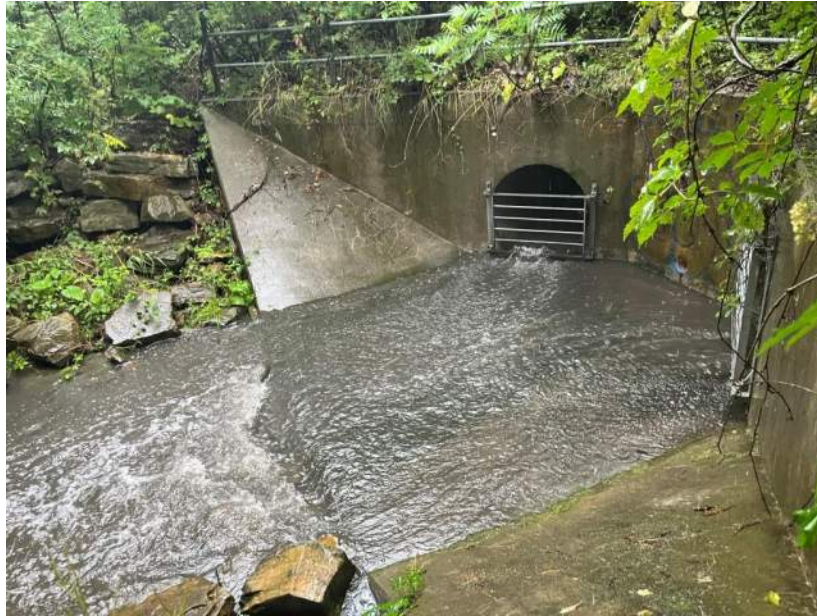
Photograph 7: Stormwater outflow into the Watts Creek tributary at Eagleson Road. Direction: Northeast
