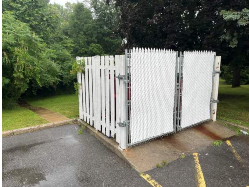
Photograph 3: Existing garbage bin enclosure to be removed. Direction: North
