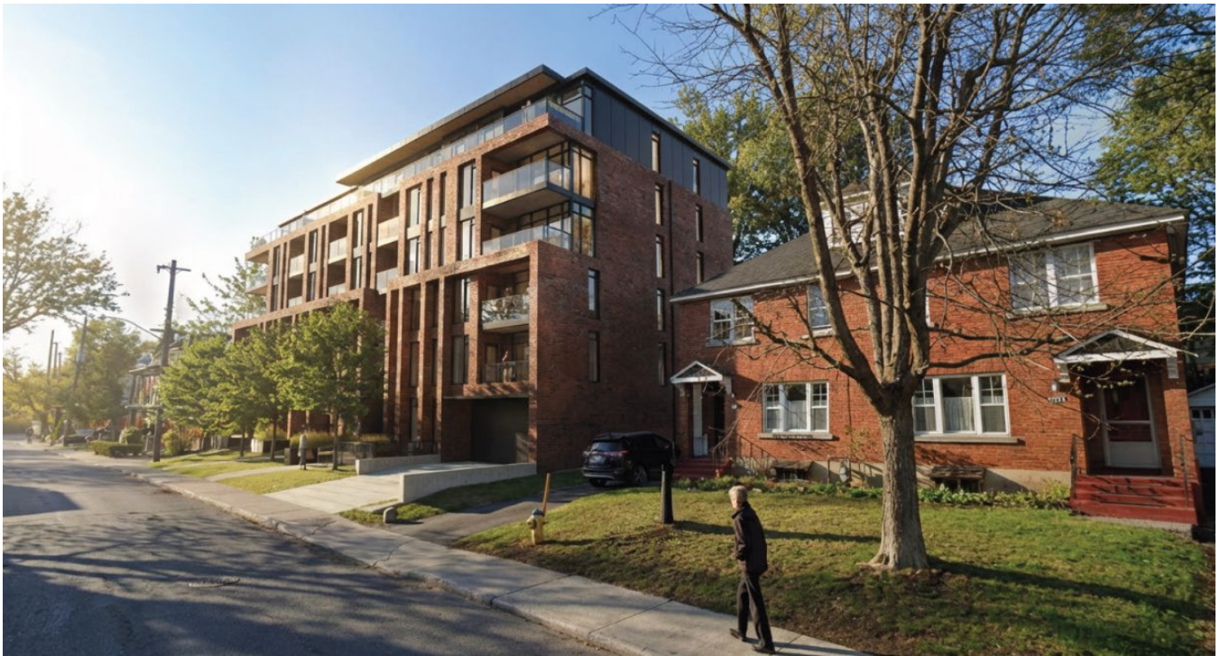
Figure 16: View from Echo Drive looking north, prepared by Project1 Studio
