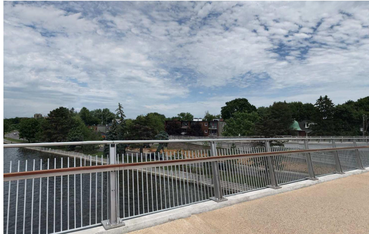
8. Looking North-East from Flora Footbridge
