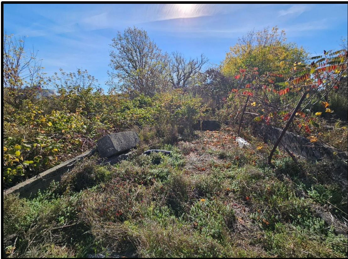
Photograph 4: View of the old foundation on the Phase I Property.
