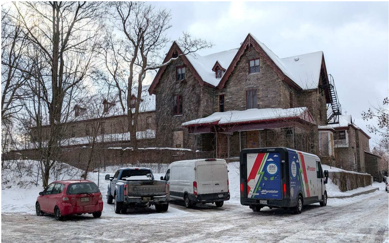
Figure 5: Northeast corner of former convent building including circa 1864-1865 Gothic Revival house on slight rise of land and circa 1913 east and north convent wings. (Heritage Studio, January 2026)
