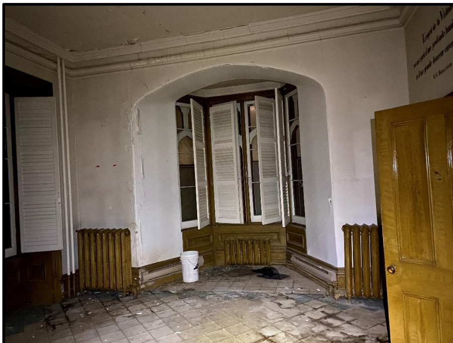
Photo 12: Room in main floor of subject building.
