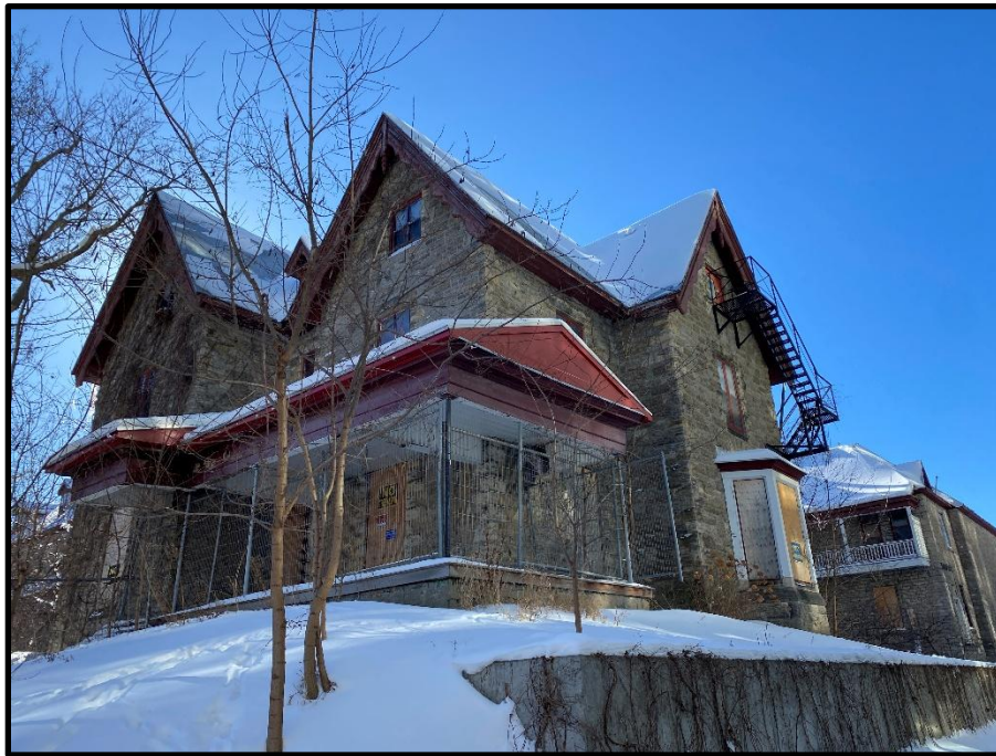
Photo 3: North east corner of the subject building.
