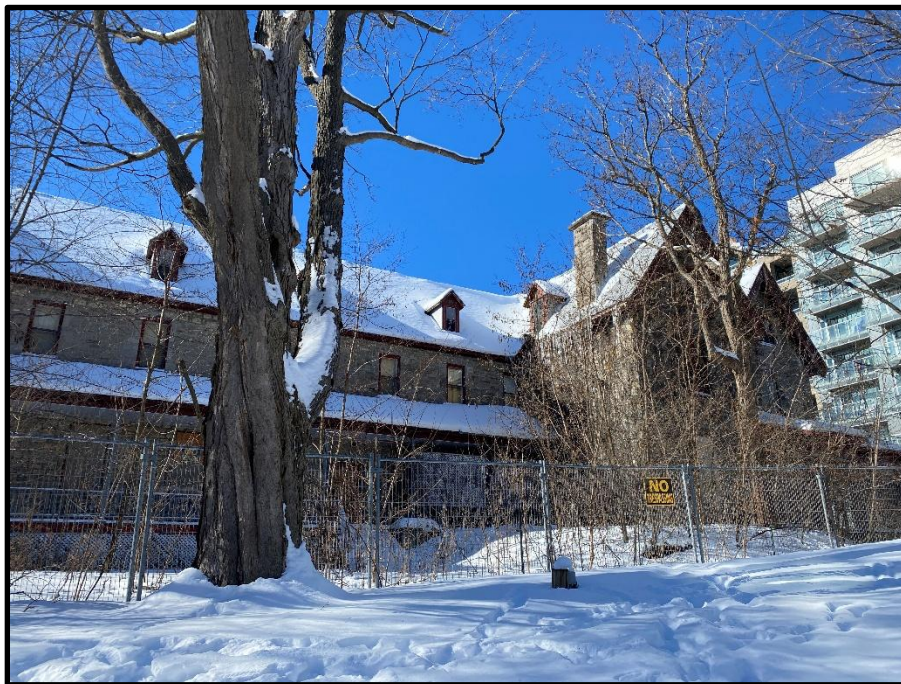
Photo 4: East side of the subject building.
