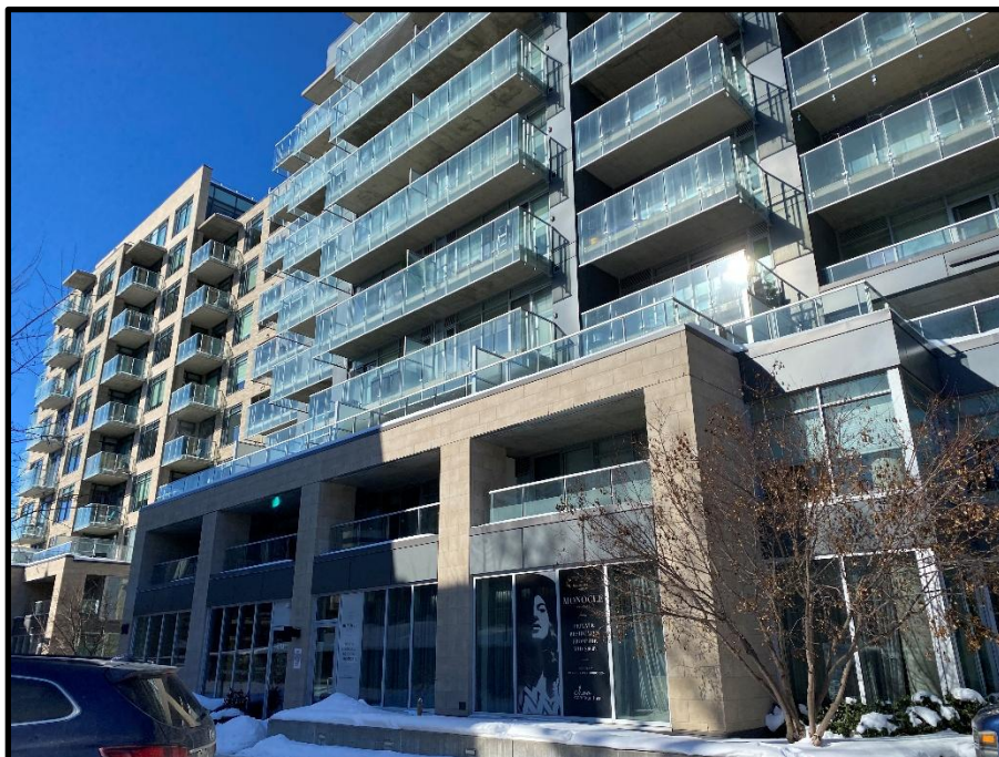
Photo 16: Surrounding properties to the north of the Phase I Property.
