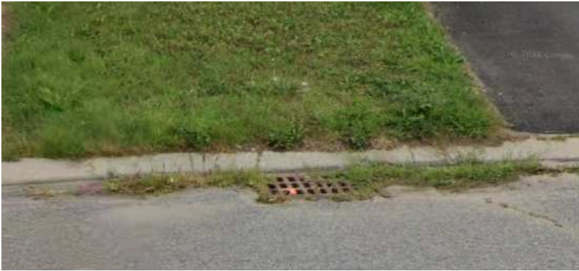
EX CB 1A - near curb of roundabout (Google Street View)
