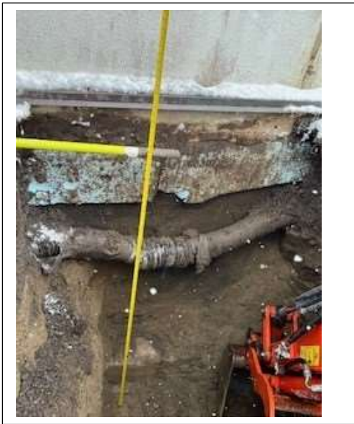
Depth from underside footing to existing grade
