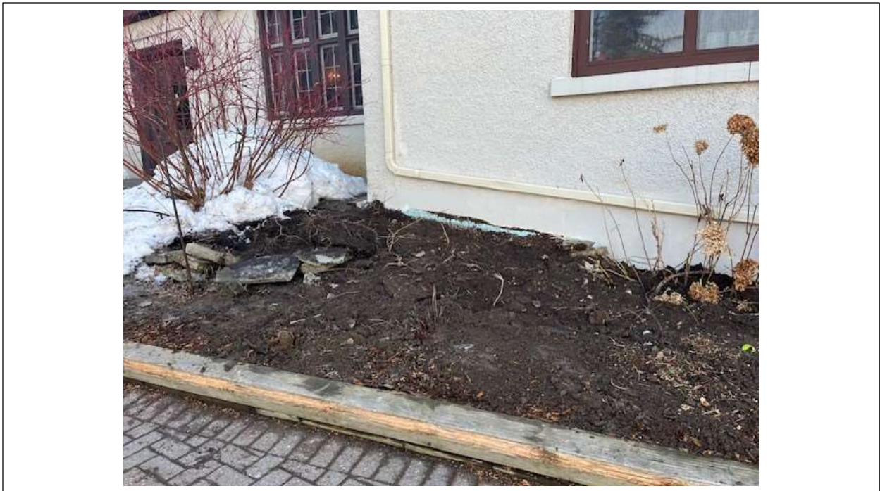
Backfilled pit location
