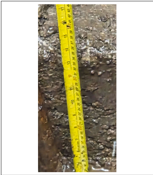
Depth from underside footing to top of footing
