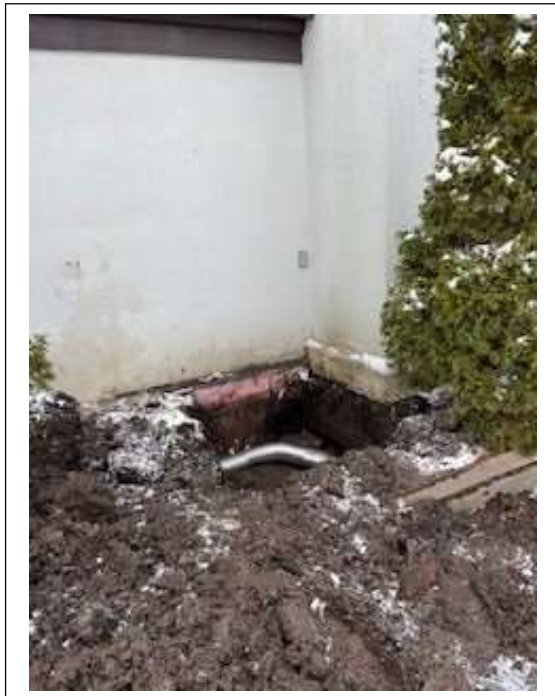
Pit Backfilled – Drain Tile Reinstated
