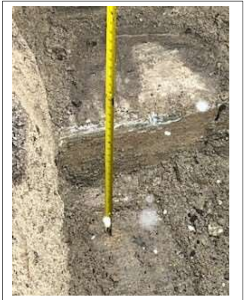
Exposed Footing & Bedrock surface
