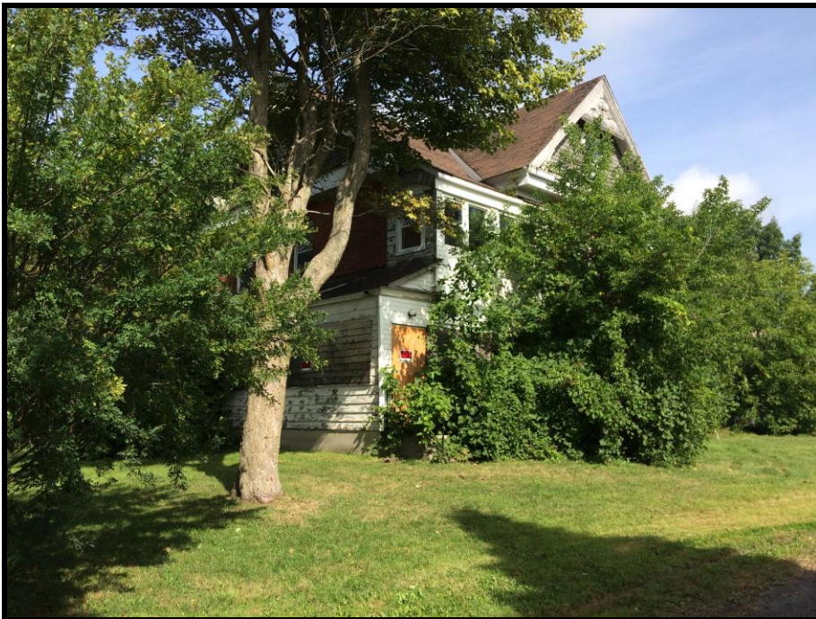
Photograph 4: View of the abandoned farmhouse, situated on 4055 Russell Road.
