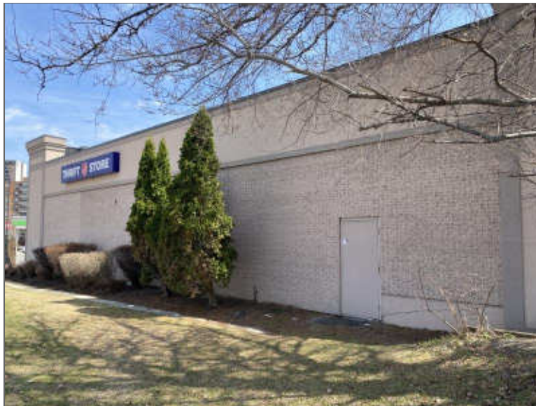
Photo 2 – View of Building A, north side, looking southeast.
