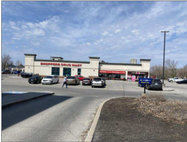
Photo 7 – Southeast corner of Site, looking north.
