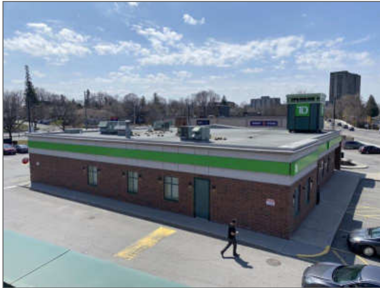
Photo 5 – View of Building B, looking eastward.
