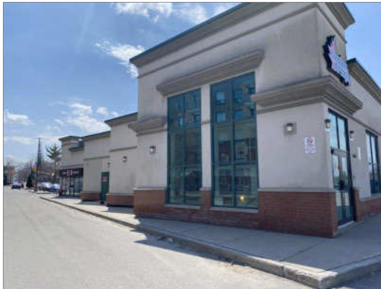
Photo 6 – View of Building C, at northwest corner- looking south.
