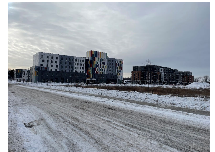
Site Photograph No. 9 • View South along Bareille-Snow Street
