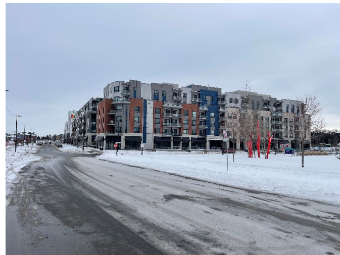
Site Photograph No. 11 • View East along Hemlock Road at Codd's Road
