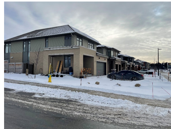
Site Photograph No. 8 • View Southeast along Bareille-Snow Street
