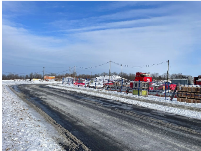
Site Photograph No. 2 • View Northeast from Codd's Road
