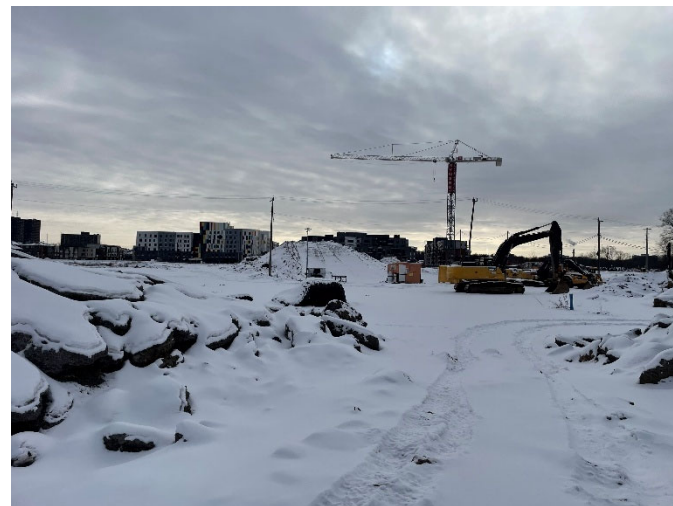
Site Photograph No. 5 • View South towards the development site
