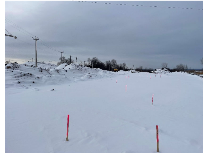
Site Photograph No. 6 • View West along future Codd's Road
