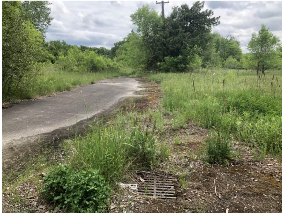
Photo 1: Typical vacant area on-Site showing former base infrastructures and old roads.
