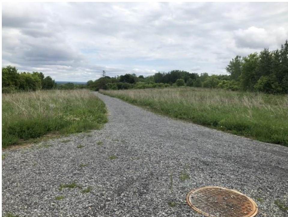
Photo 4: Vacant lands adjacent west of the Site with recently installed sewer lines.
