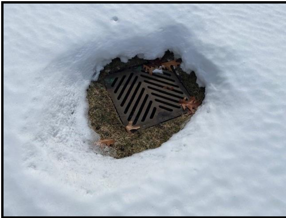
Photograph 6: View of the catch basin located in the central portion of the Phase I Property
