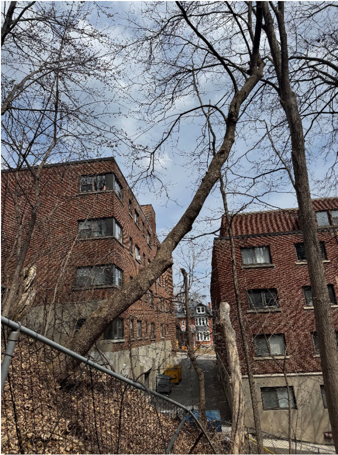
Photo 1: Tree 27, Manitoba maple on adjacent property that should be removed due to the potential for failure on subject property
