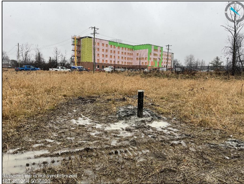
Monitoring well observed in the south portion of the Site
